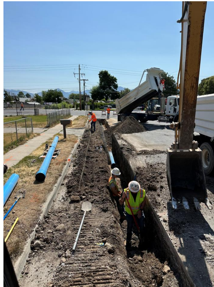
Cherrywood Waterline – GHID crew trenching, laying pipe and backfilling
