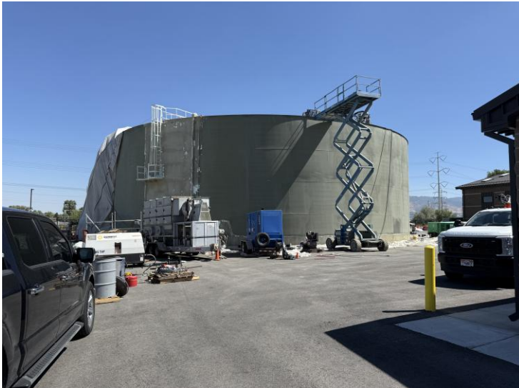
South End of Acord Reservoir Prepped for Coating
