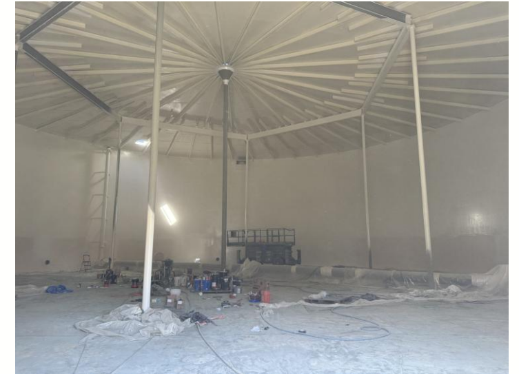
Completed Interior of Acord Reservoir
