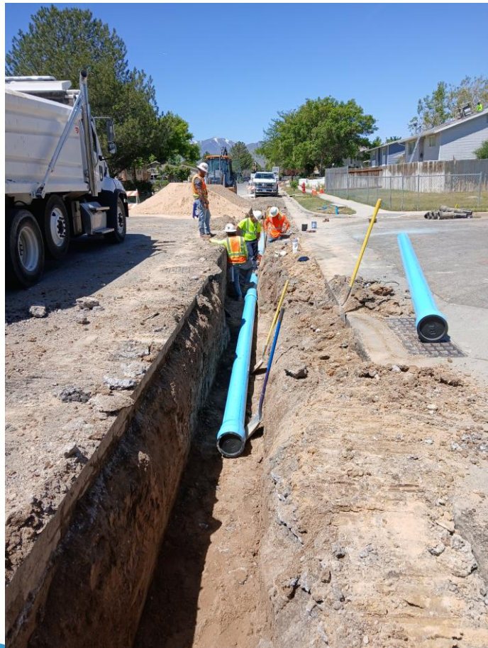
Cherrywood Waterline – GHID crew trenching, laying pipe and backfilling
