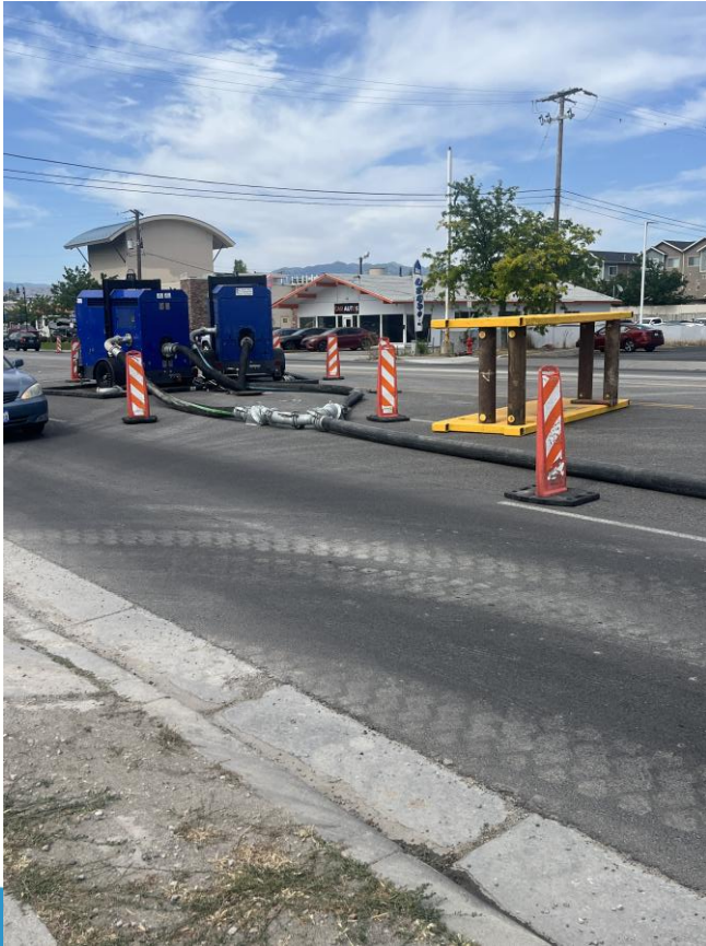
Redwood Road Bypass Setup
