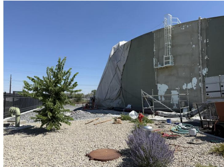
Sand Blasting and Hazardous Waste Mitigation on West Side of Acord Reservoir
