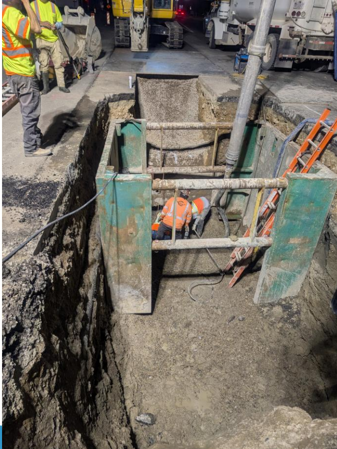
3500 South Flowable Fill Placement
