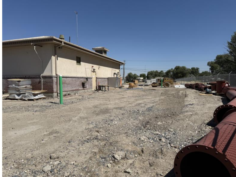
East Side of Well No. 16 Where New Sewer and Storm Sewer Is Installed
