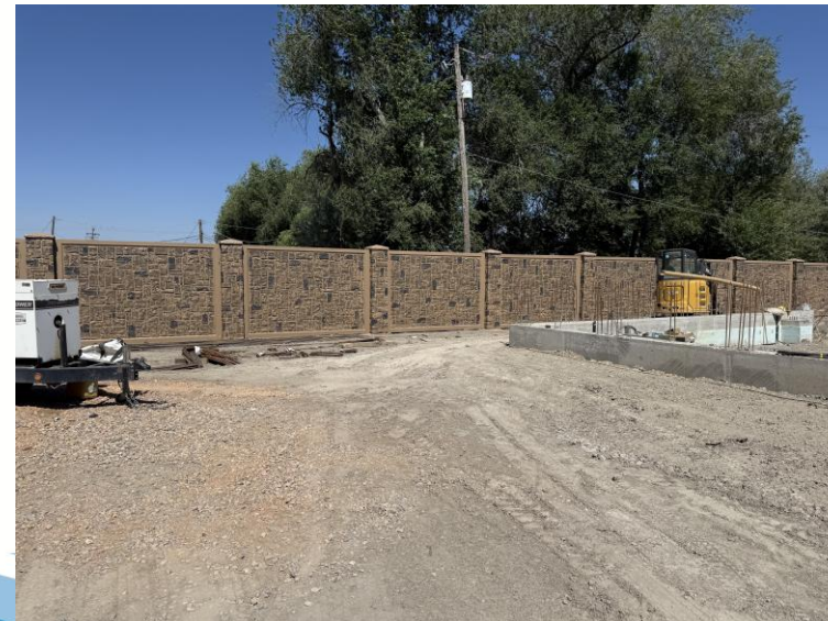
Completed Fencing on West Side of Anderson WTP Project Site
