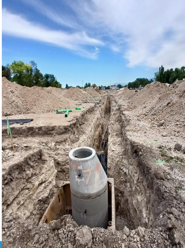
Manhole and sewer trench
