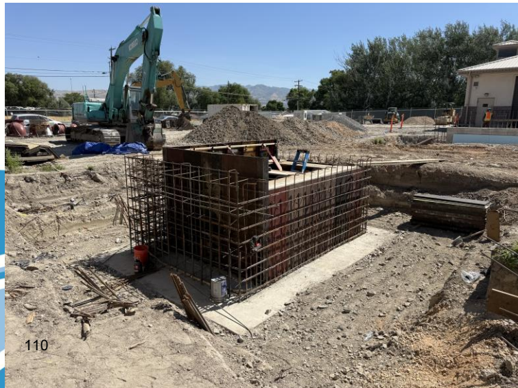
Transmission Line Vault on North Side of the Future Anderson WTP Building
