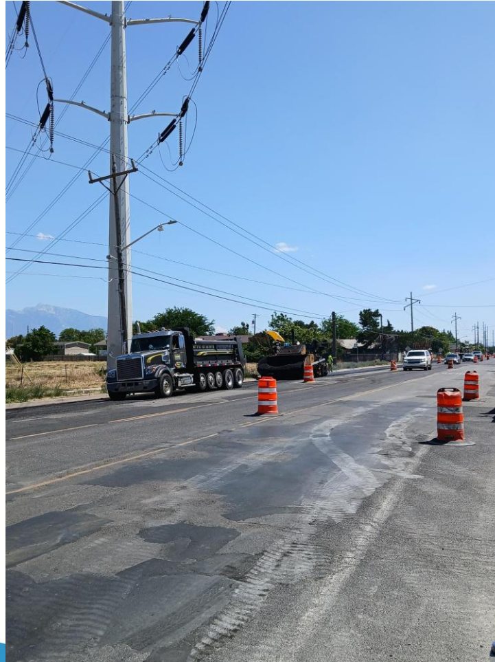
Lowering and raising manholes and valves along roadway
