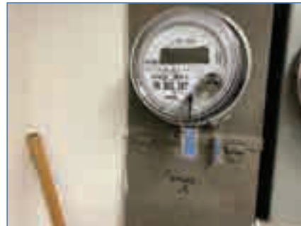
Exhibit 2 – Service A meter with error message E01
