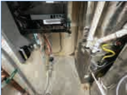
Exhibit 12 - Furnace, duct, and pipes in front of telecom rack
