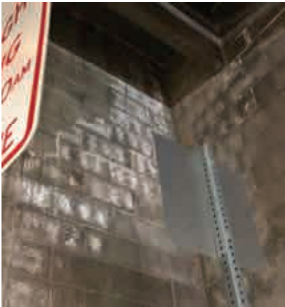
Photo #4 – Moisture Infiltration in CMU Walls
