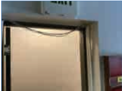
Exhibit 15 - Exposed cables above doorway.
