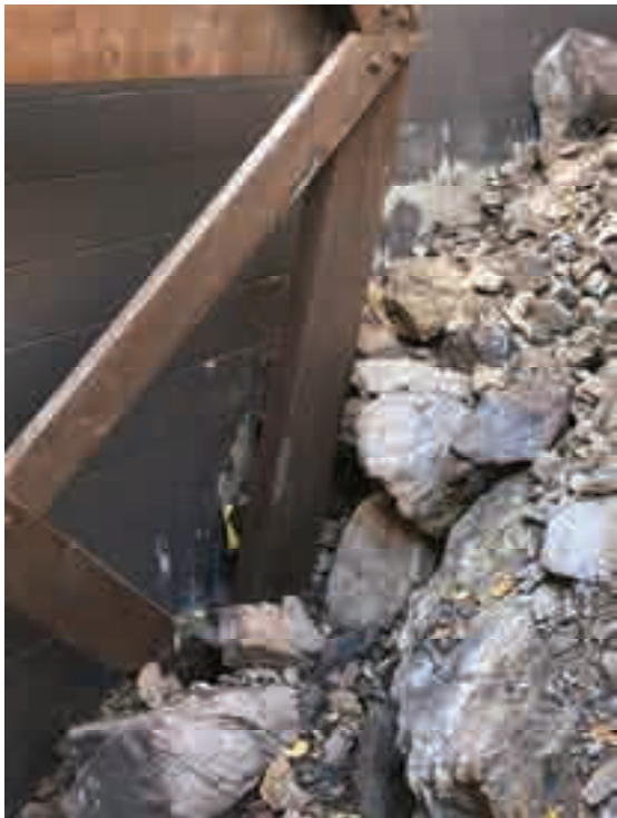
Photo #5 – Rock Fall Damage to Framed Addition Base
