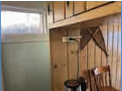
Exhibit 9 – Existing wiring devices and surface raceway
