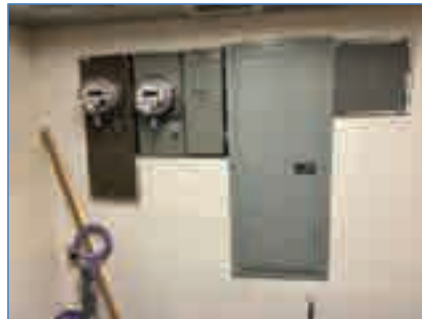
Exhibit 1 – Service A and B meters and panelboard B
