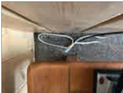
Exhibit 15 – Coax cable punched through floor
