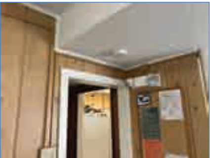
Exhibit 12 –Emergency bug eye and toggle switch
