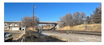
Constructed in 1985 and spanning approximately 120 feet, this bridge spans four sets of railroad tracks on the north border of Clearfield. It has a single travel lane in either direction and carried an average of 9,000 vehicles per day in 2024. There is a sidewalk on the north side of the bridge. Based on the most recent inspection, this bridge is currently in fair condition. As this bridge was
