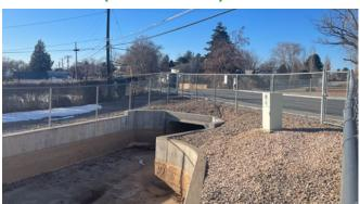
This bridge spans the Weber Davis Canal on the east side of Clearfield. This bridge was built in 1965. It has a single travel lane in either direction and sidewalks on both the north and south sides. This bridge was reconstructed as a box culvert in 2023. As it was reconstructed after 2000, the anticipated design life is 75 years. Thus, the anticipated timeline for this culvert to be replaced is sometime between 2090 and 2095.
