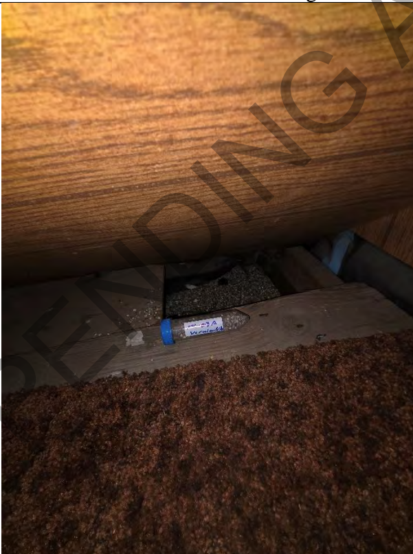
176 – 03A Vermiculite Insulation
