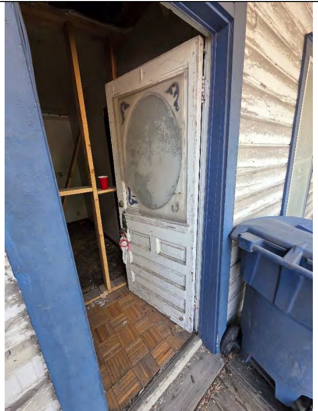
Lead exterior door, siding and door frame
