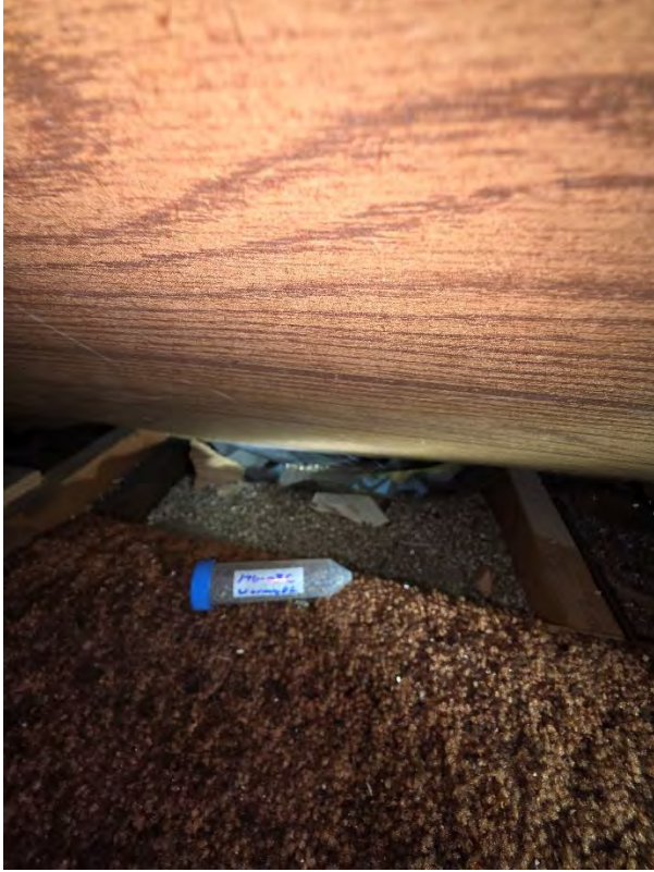
176 – 03C Vermiculite Insulation
