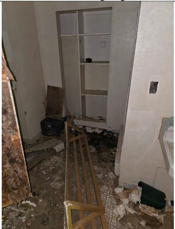
Basement South Apartment bathroom
