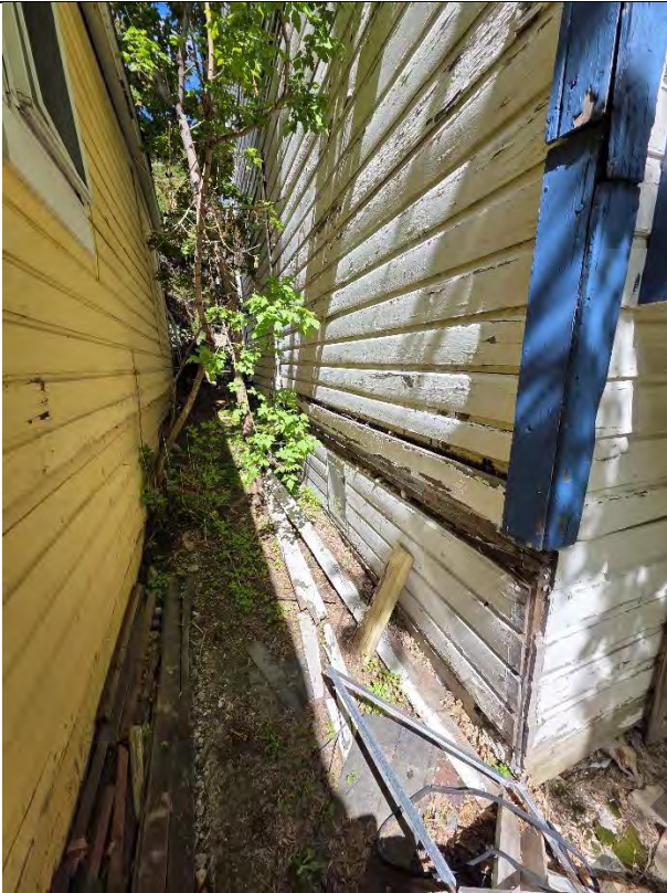
Lead exterior siding and trim
