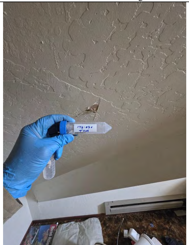
176 – 02C Textured Wall/Ceiling Material
