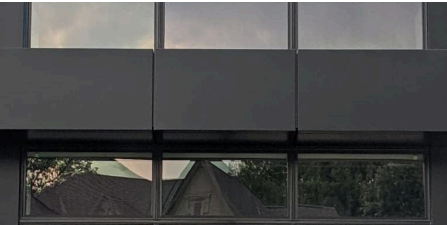
6 STEEL AWNING FACED WITH ARCHITECTURAL PANELS - CLOSED CONTRACTOR BLACK POWDER COAT
