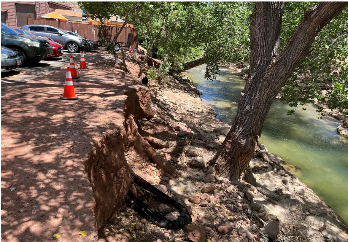
**Figure 5** – July 12, 2023. Right bank of North Fork Virgin River downstream of project area, looking upstream. A vertical cut bank has formed adjacent to the parking lot downstream of the proposed facility.
