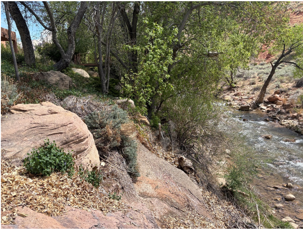
Figure 7 – April 17, 2025. Looking upstream partway up the right (west) overbank of the North Fork of the Virgin River. The apron of grout is visible in the forefront of the image. This grout is present between the lower tiers of keyed in boulders and appears to be between 2 and 6 inches thick. The overbank adjacent to the Custer Residence is heavily vegetated.
