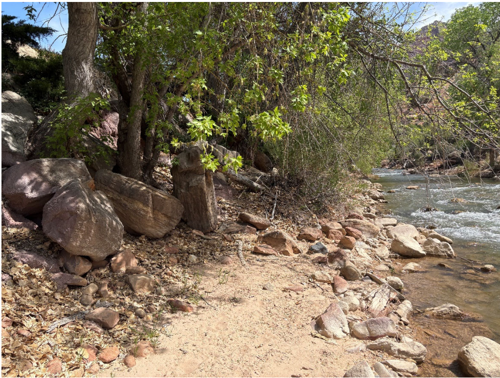
Figure 5 – April 17, 2025. Looking upstream along the west (right) overbank adjacent to Parcel S-CSD-4. The bank armoring that was previously completed plays a significant role in the stability of this section of streambank. The grout located around some of the larger cottonwoods has limited erosion, preventing undercutting from occurring.
