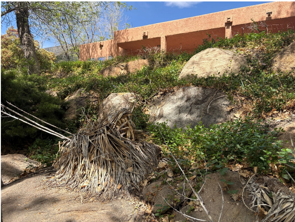
Figure 8 – April 17, 2025. Image of the keyed boulders and vegetation along the right (west) overbank of the North Fork of the Virgin River adjacent to the residential structure.
