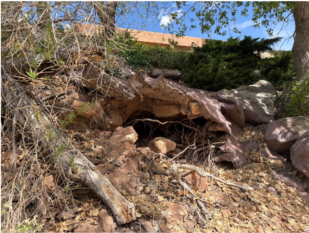
Figure 9 – April 17, 2025. Image of damage to a grouted section of the streambank armoring. It appears that the damage was caused by either a large mature cottonwood falling into the river, or a large boulder being displaced. The damage is approximately 4' wide and 3' tall.
