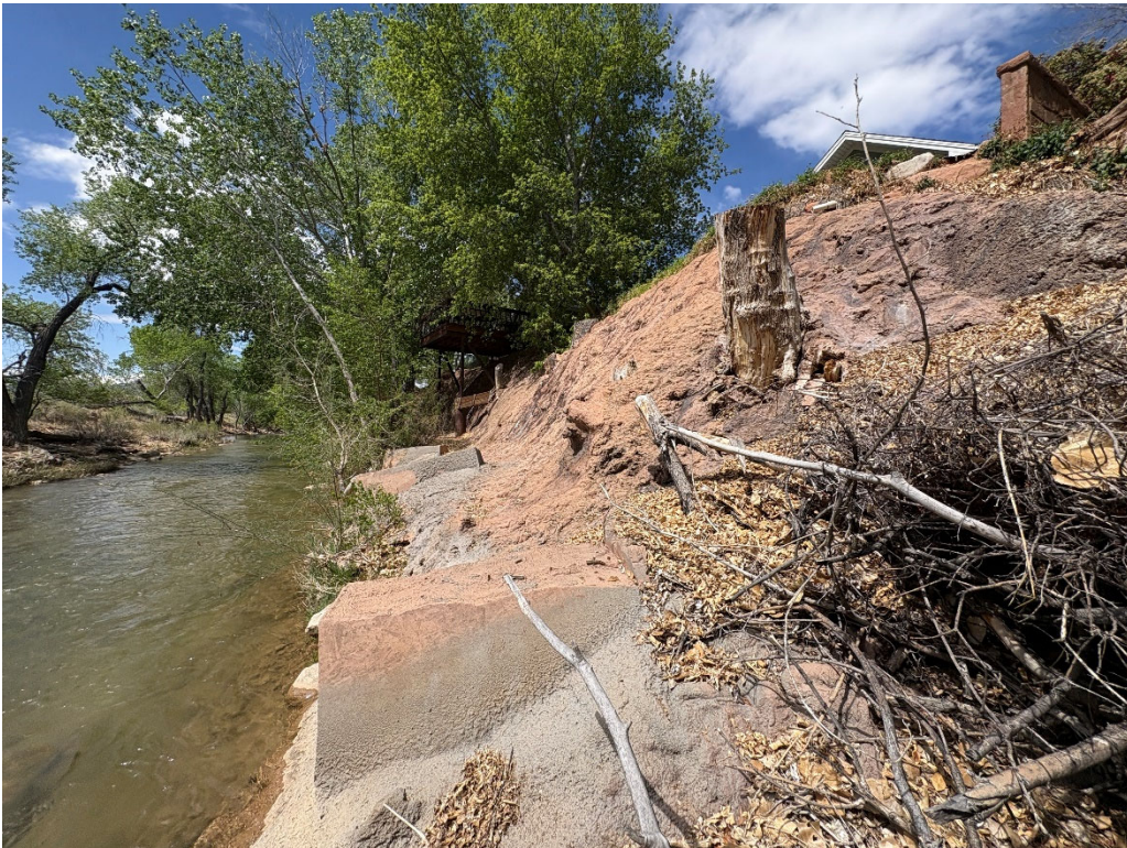
Figure 10 – April 17, 2025. Looking downstream along the right (west) overbank of the North Fork of the River at the grouted apron adjacent to the property downstream of Parcel S-CSD-4. Many of the cottonwood trees that had grout placed around them have decayed, leaving holes in the structure. Three "stream barbs" are present adjacent to the waters edge, which will help push high velocity flows away from the bank. The presence of this bank armoring provides limited protection to the proposed improvements by providing stability to the main channels location.
