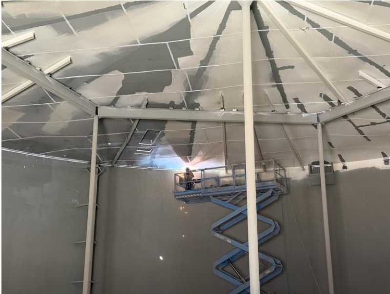
Acord Reservoir roof rafter installation
