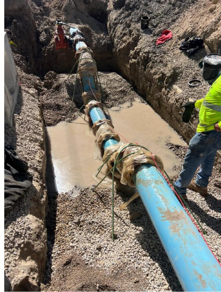
8" water main loop for storm drain conflict
