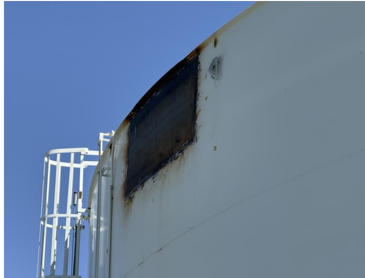
Acord Reservoir structural repair on Southwest corner
