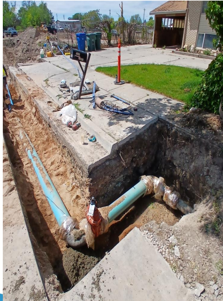
8" water main tie-in with thrust blocks and wax wrap
