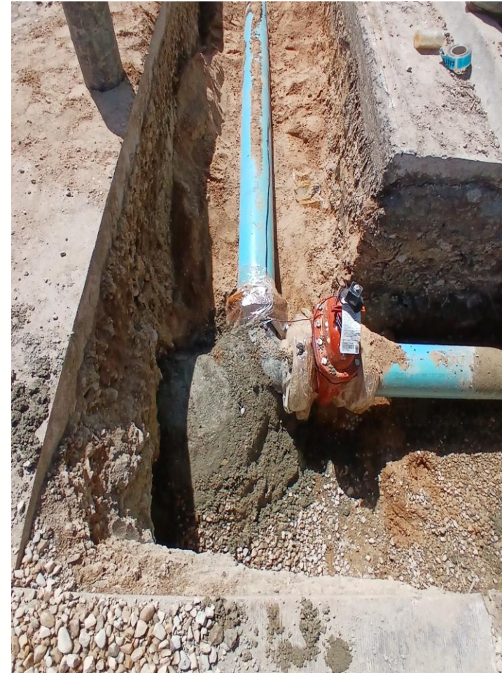
8" water main tie-in with thrust blocks and wax wrap
