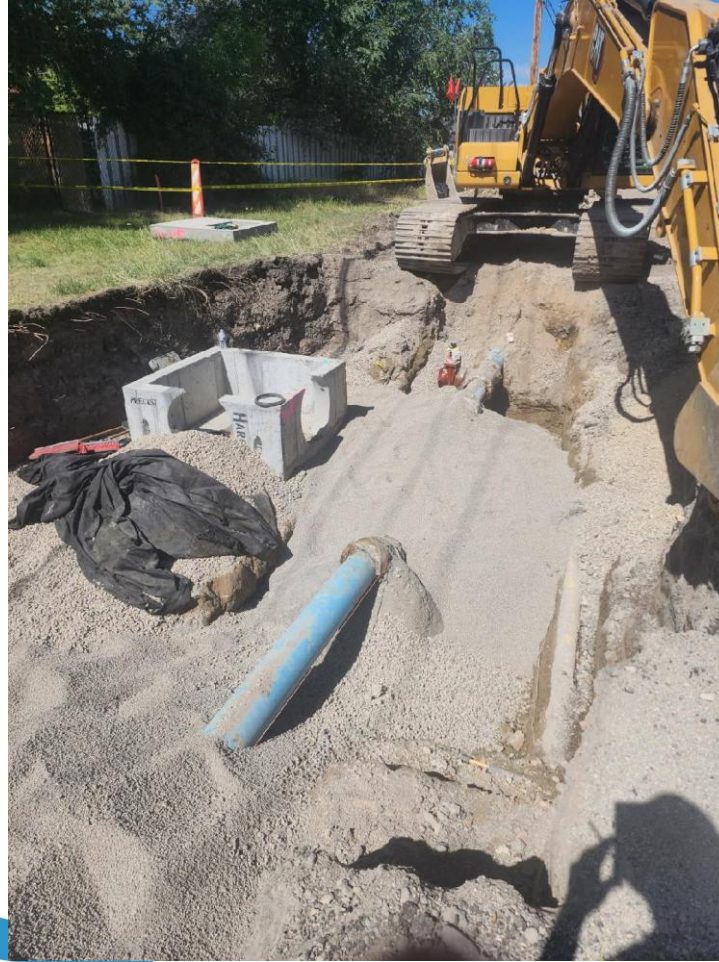
8" water main loop for storm drain conflict
