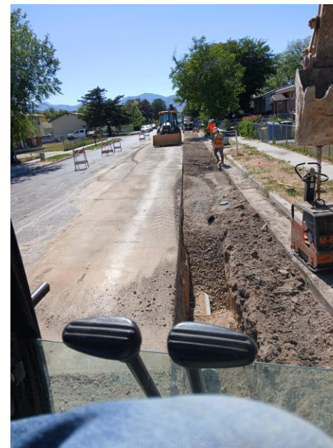
Cherrywood Waterline – Backfilling trench
