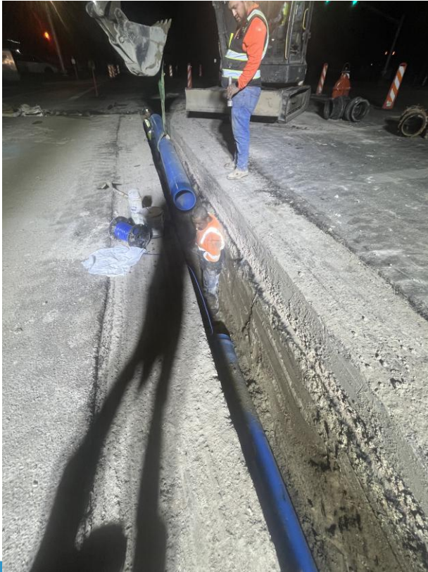
Redwood Road 12-inch Waterline Installation
