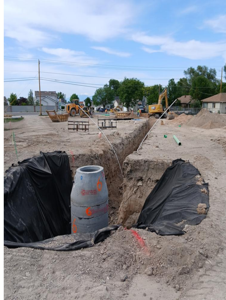
Manhole installation
