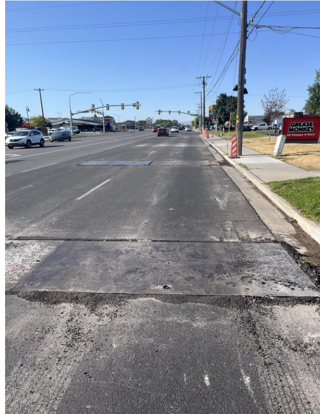
Redwood Road Roadway Trench Repairs
