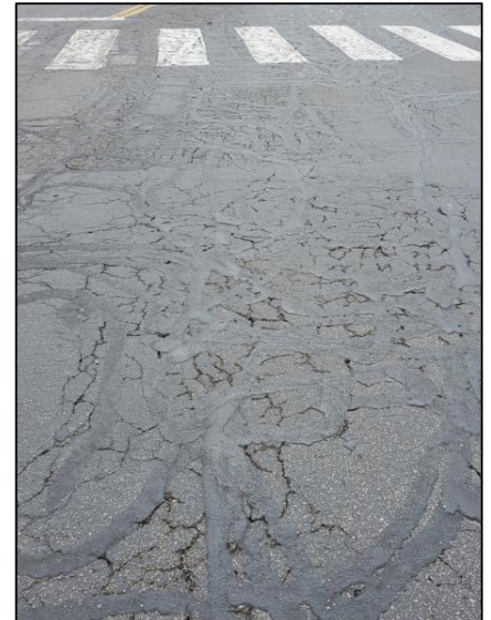
4200 South 3900 West- No cross slope or crown, which results in hazardous ponding at times and ponding in the crosswalk.
