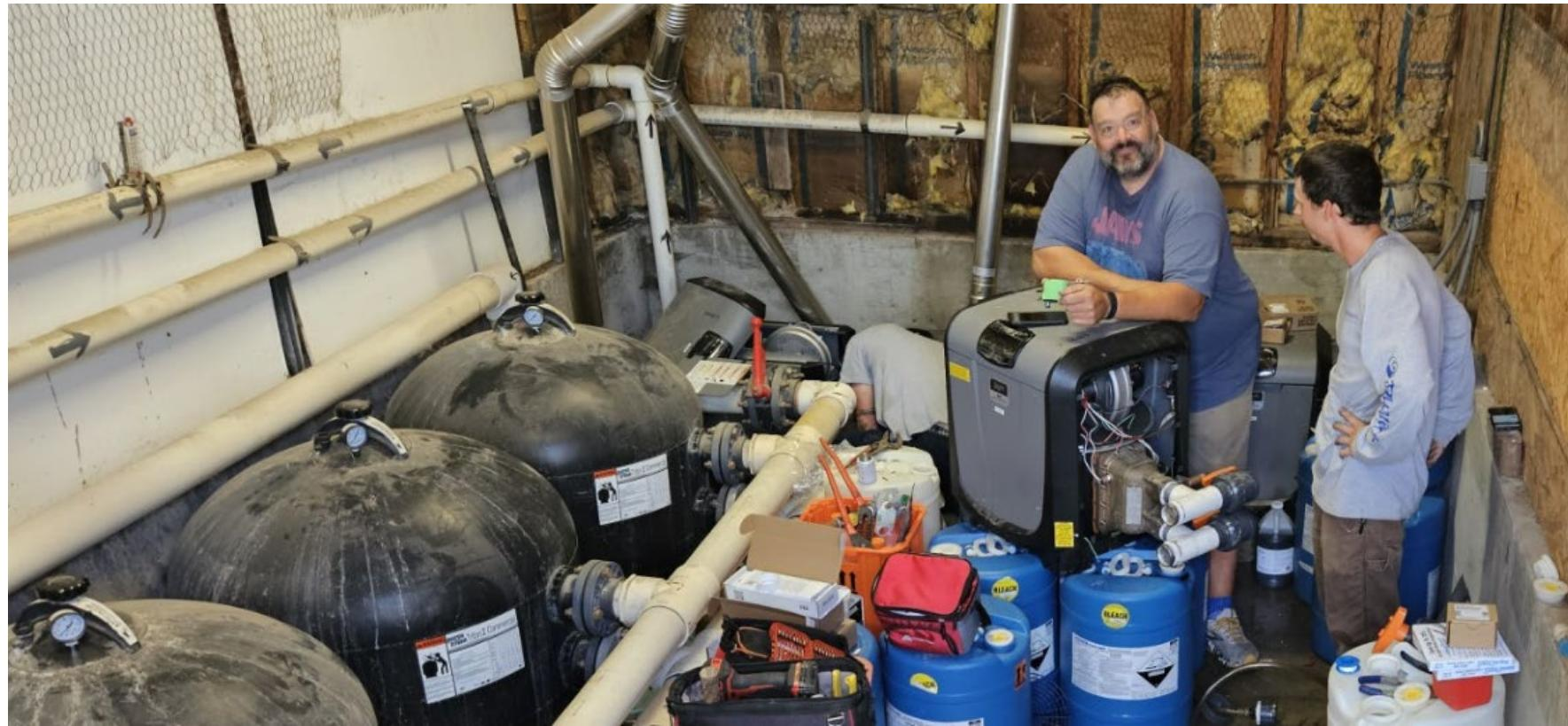
When the boilers were restarted, it was determined there was insufficient flow, which was largely responsible for the issue. The circled part is a 2001 flow controller, which should have been replaced at the time of the installation.
