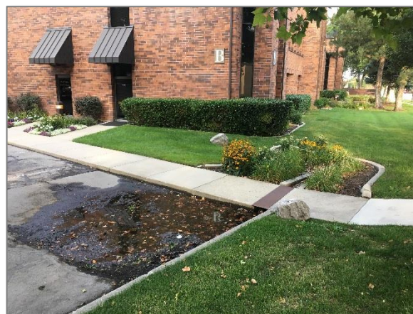
Figure 11: Standing water after a rain event at a bioretention BMP.
