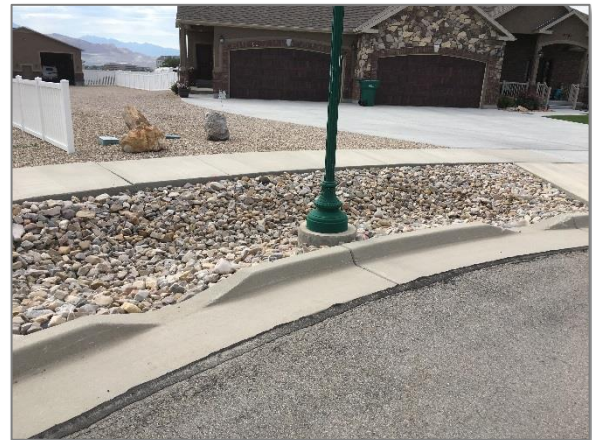
Figure 8: Curb cuts to a rock lined swale.
