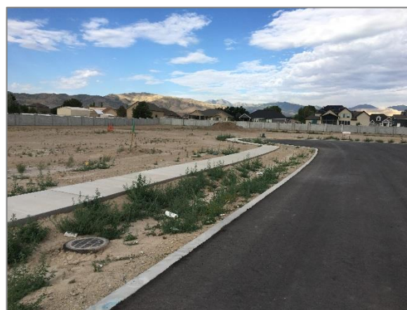
Figure 12: A vegetated swale that will provide pretreatment for a dry well.
