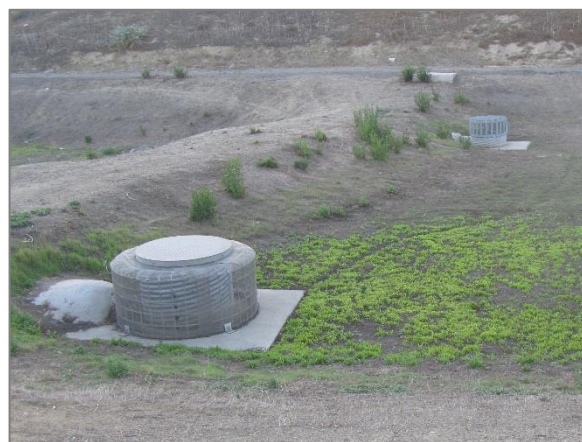
Figure 4: Multi-stage overflow outlet with trash screen
