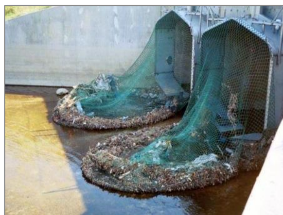
Figure 5: End-of-pipe trash netting
