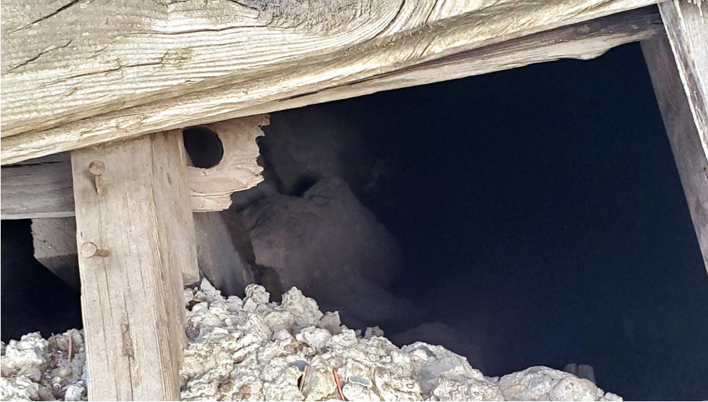
PHOTO #2 - FRONT DECK/ FOUNDATION STRUCTURE
