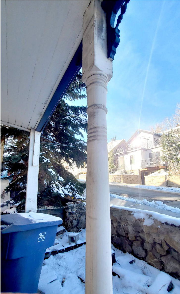
Back of Front Deck Post
