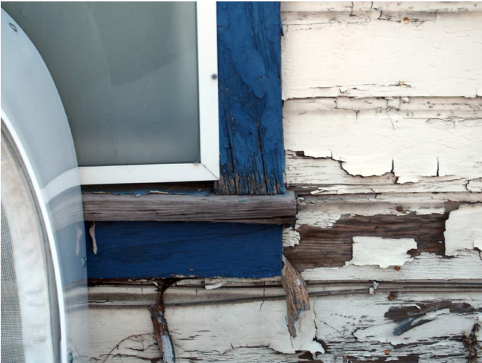
Window Trim at West Elevation
