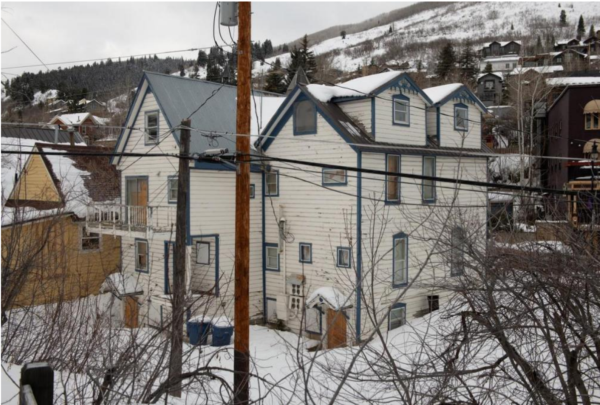
176 Main Street looking Southeast
