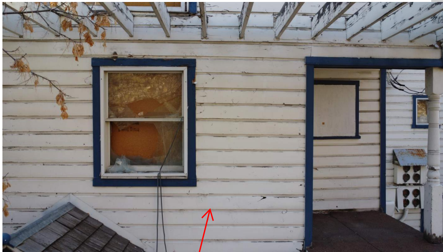
Newer Siding on more recent addition to 1907 structure
