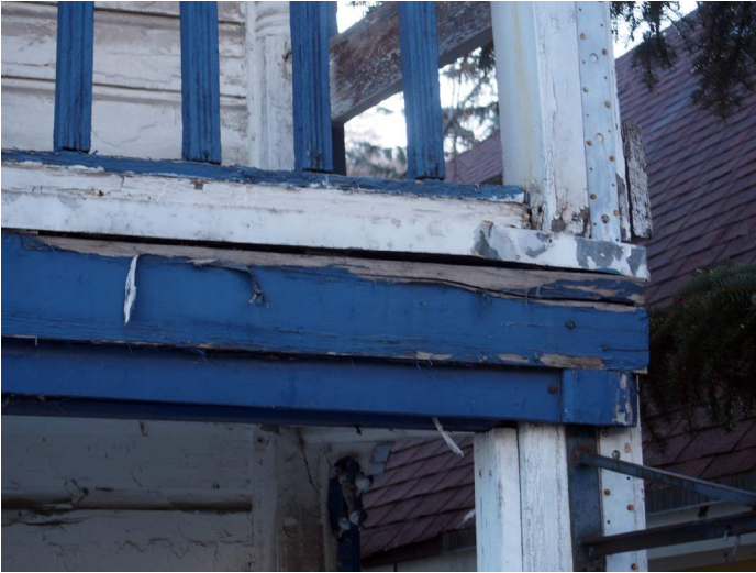
Trim at Front Porch SW corner
