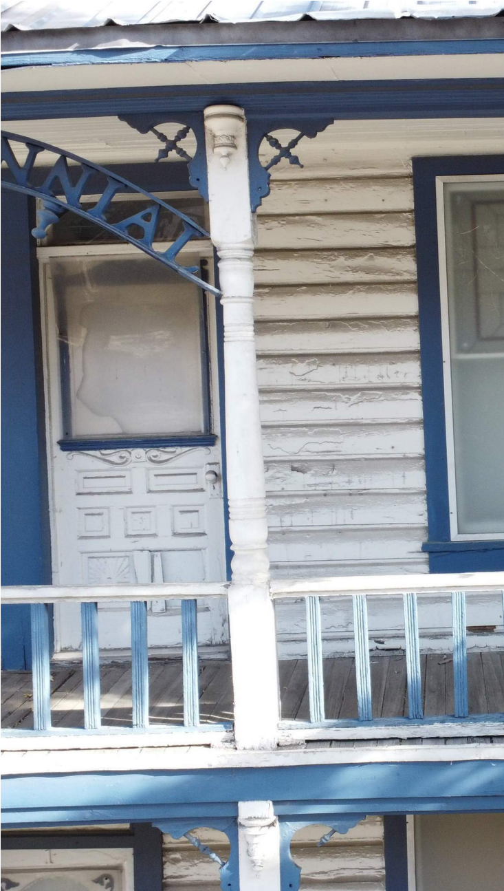
Upper Front Deck post
