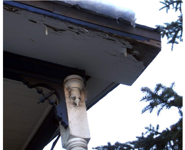
Upper Front Deck corner post
