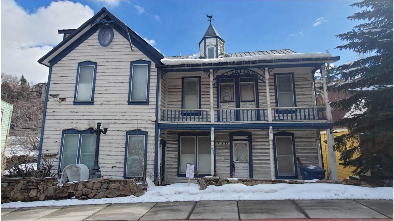
PHOTO #1 - ENTRY WALL AND WALKWAY
