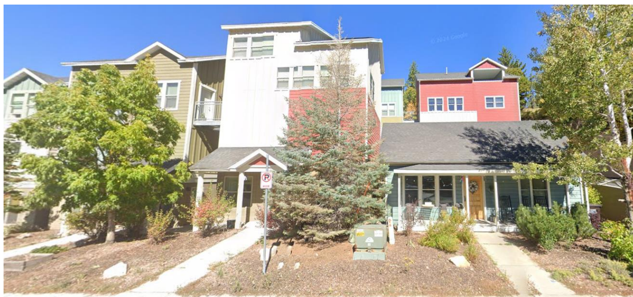
Figure 2: 555 Deer Valley Drive, Unit #10 is the Significant Historic Structure on the far right, painted blue
