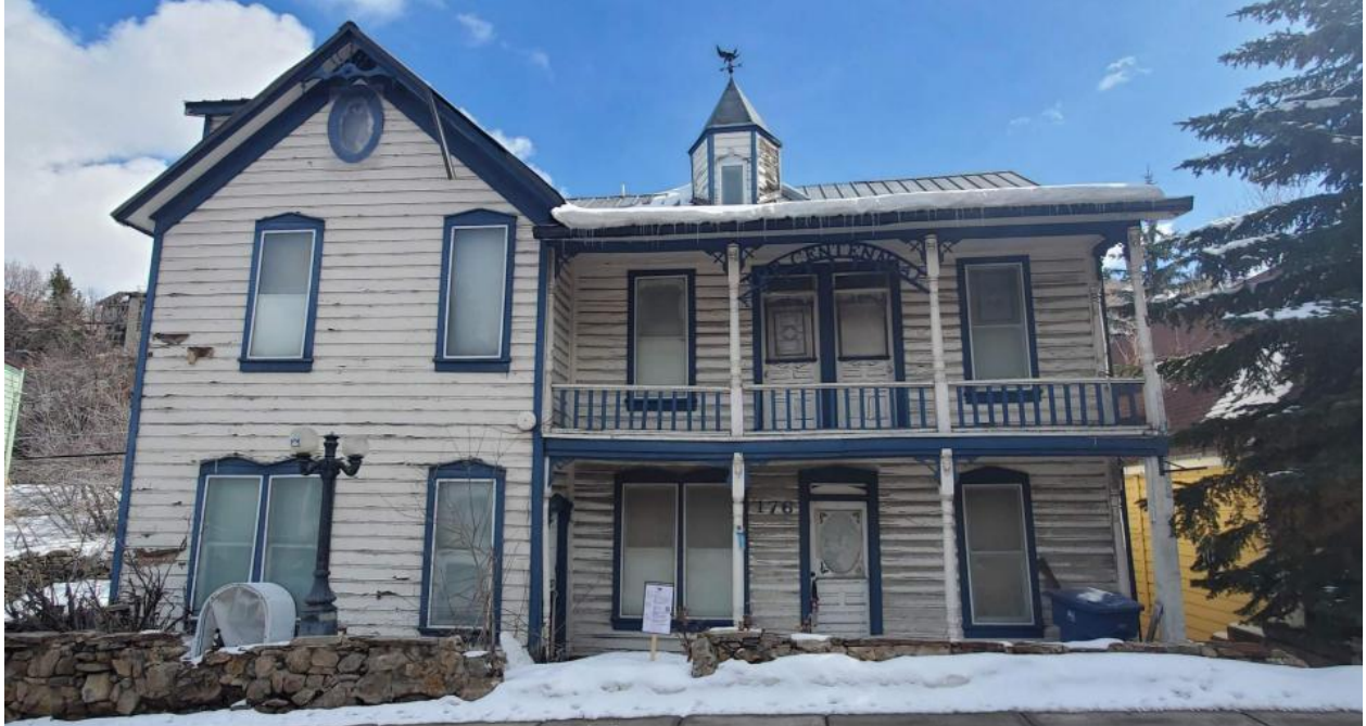
176 Main Street viewed from Main Street
