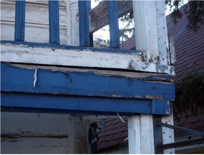
Trim at Front Porch SW corner
