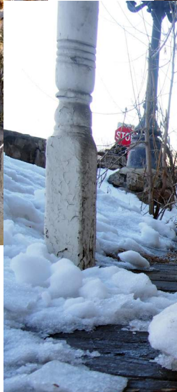
Base of Front Porch Post
