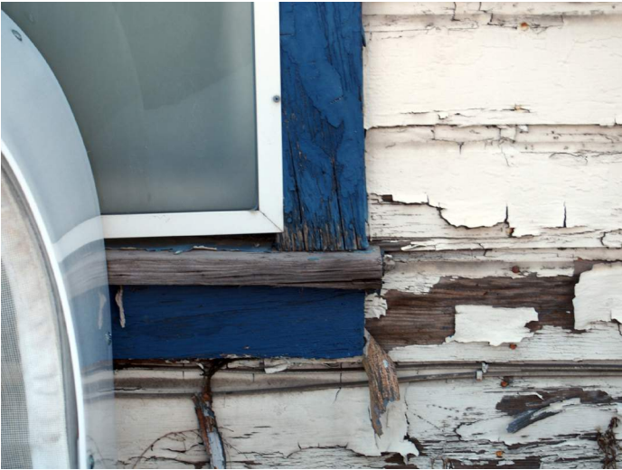
Window Trim at West Elevation
