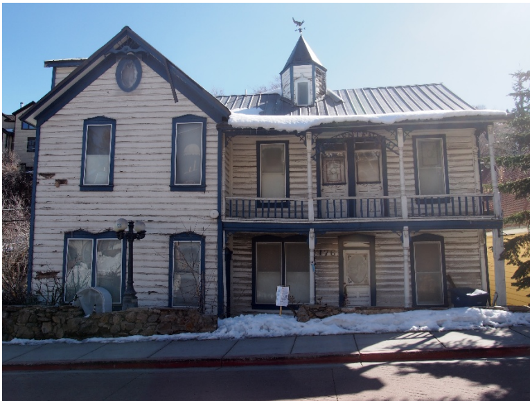
Figure 2- Concave Roof/Floor View
