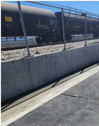
UDOT Retaining Wall Filled In
