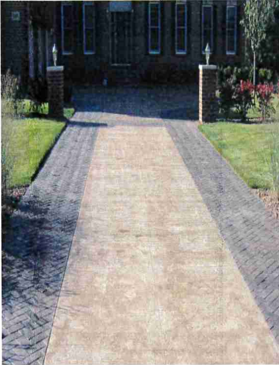
Stamped concrete. Photo courtesy of Todd's Services.
