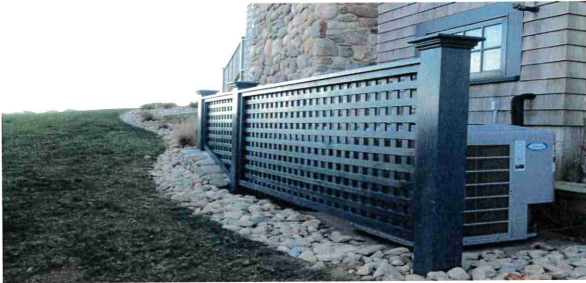
Example of ground equipment screening. Photo credit to Pinterest.
