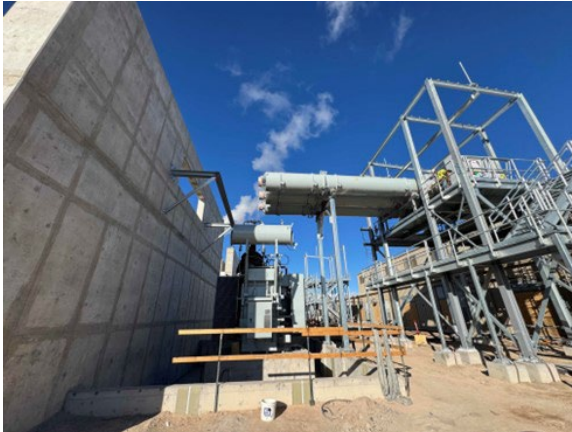
IPB Duct Gen-GCB-XFMR 51
