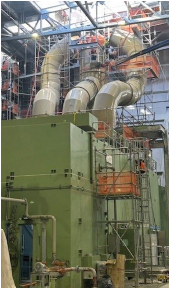
Units 3 Turbine Exhaust Piping
