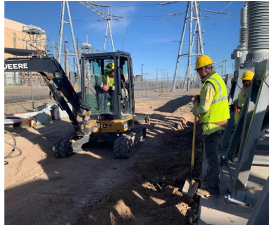
Grading Clean Up and Yard Rock Installation
