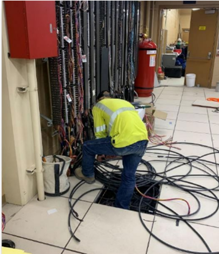
Removal/Cleanup of Old Cable in Relay House
