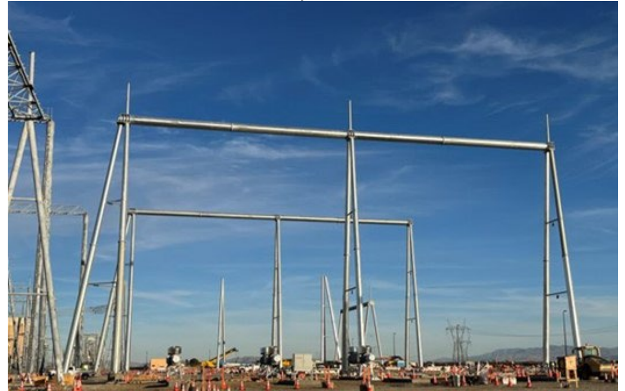
Bay 1 and 2 108' A-Frame Bridge Section completed
