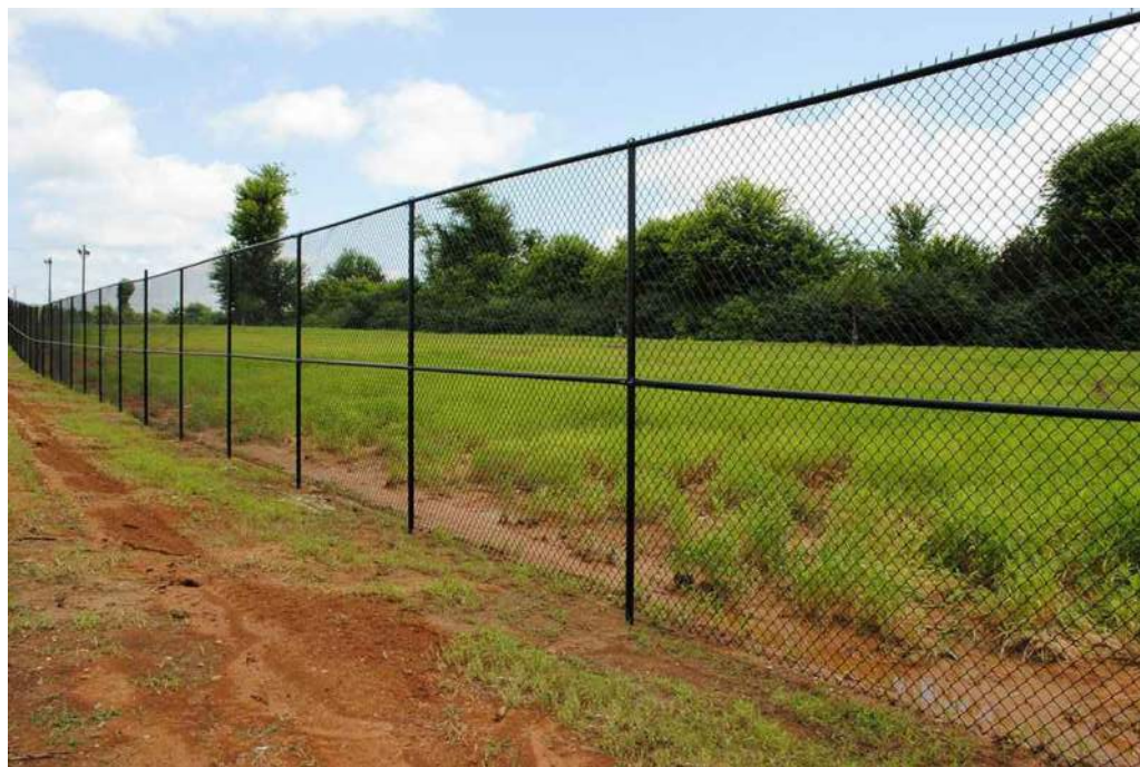
6 FT HIGH PRECAST CONCRETE FENCING
