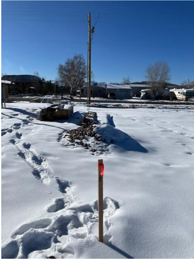
Survey Marker 1002 Centerline of Spring Hollow Access
