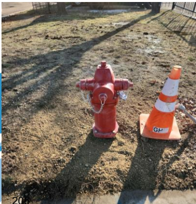
New hydrant @ 4765 W 3500 S
