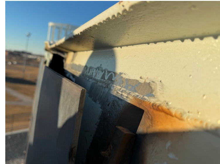
Top Portion of Reservoir Prepared for Welding
