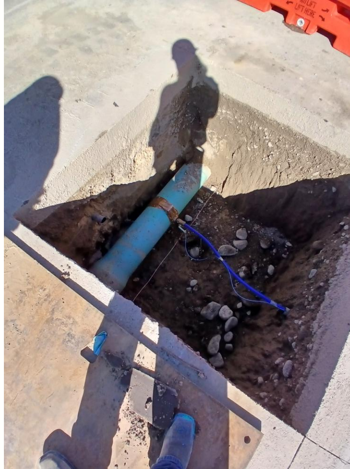
1" water lateral connection on GHID 12" PVC water main
