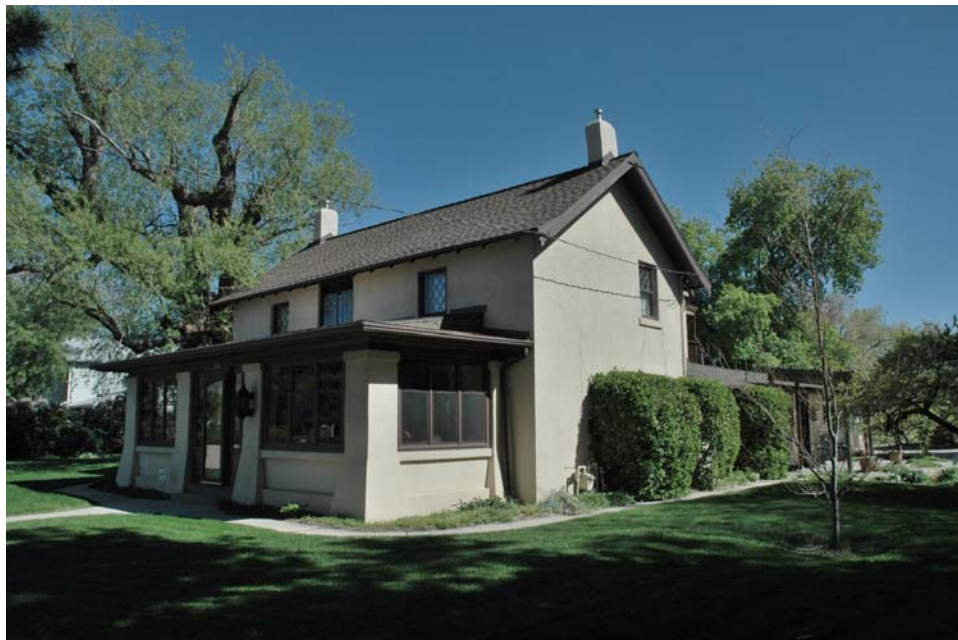
Photograph 3 of 9 North and west elevations of Bradford House. Camera facing southeast.
