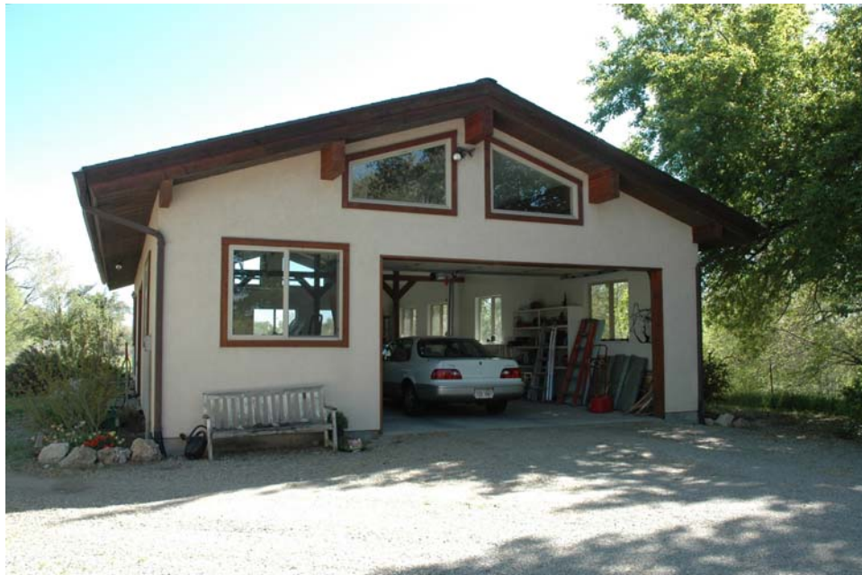
Photograph 6 of 9 North elevation of garage. Camera facing south.
