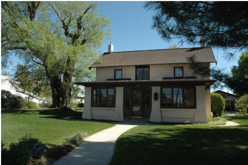
Photograph 1 of 9 View of site and north elevation of Bradford House. Camera facing south.
