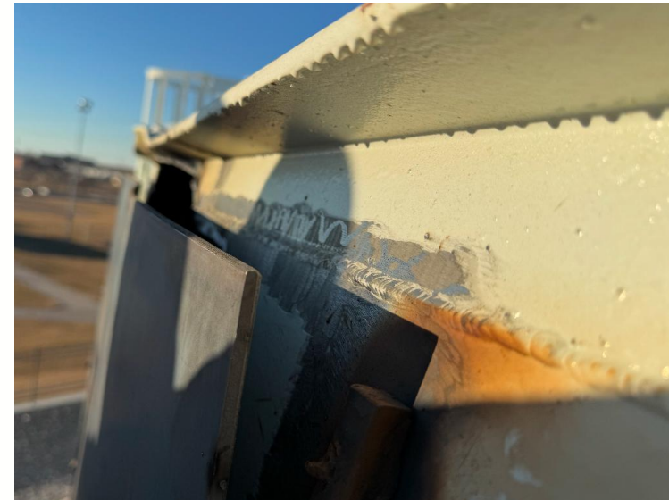
Top Portion of Reservoir Prepared for Welding
