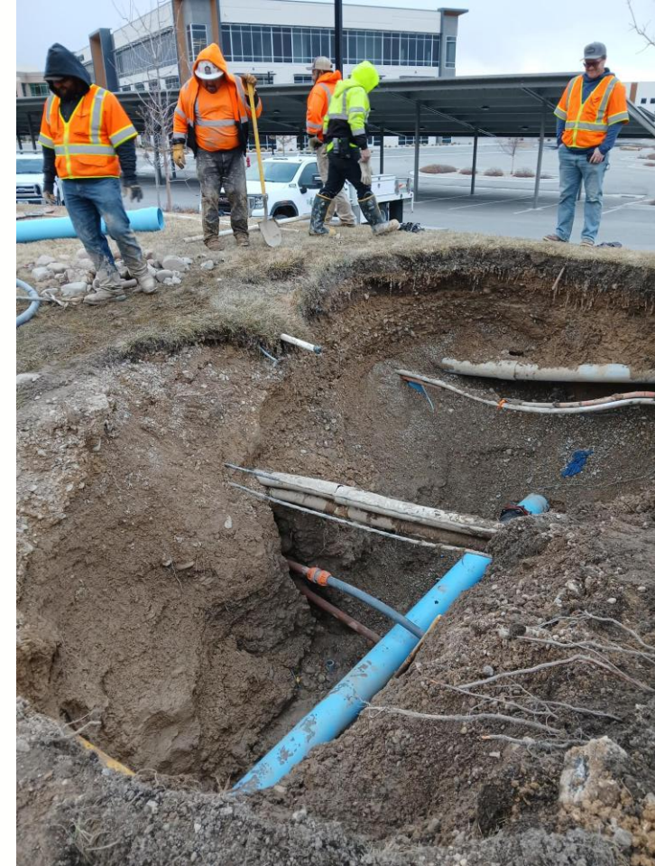
8" fire line repair
