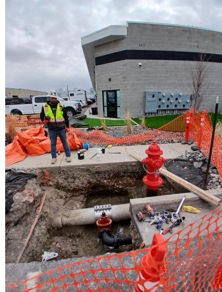
Fire hydrant installed on GHID 12" AC water main
