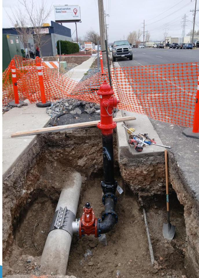
Fire hydrant installed on GHID 12" AC water main
