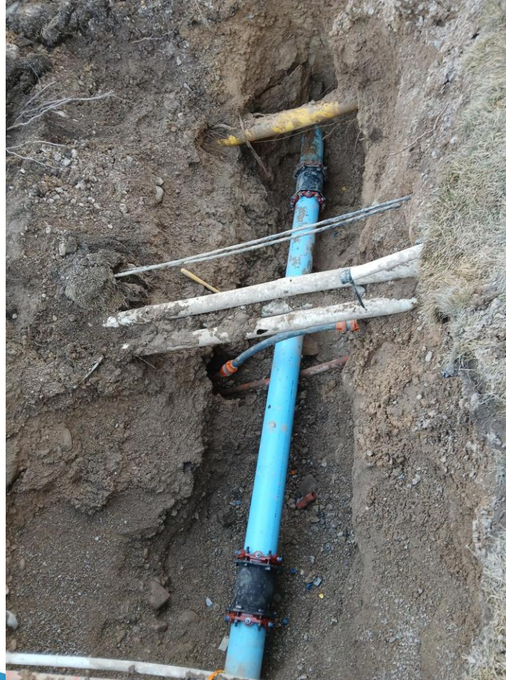
8" fire line repair
