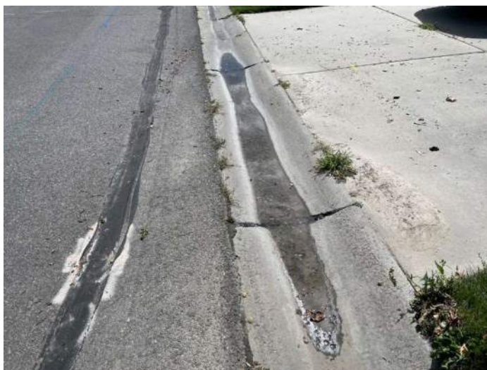
Figure 2-1: Common Gutter Style in White City
