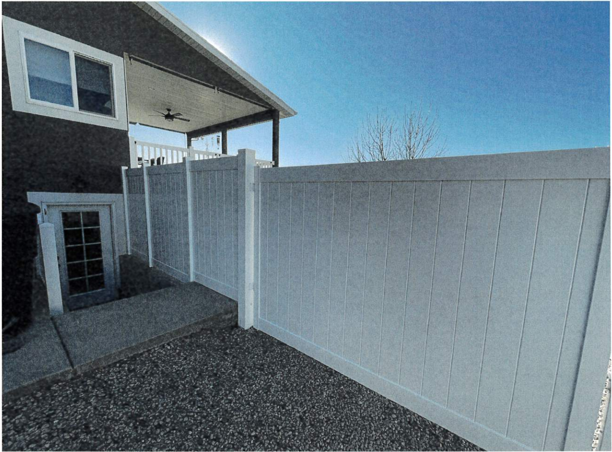
Air BnB door access (Left side of image). Locked gate inaccessible for guests. Parking available in front of this gate (Referencing the image above).
