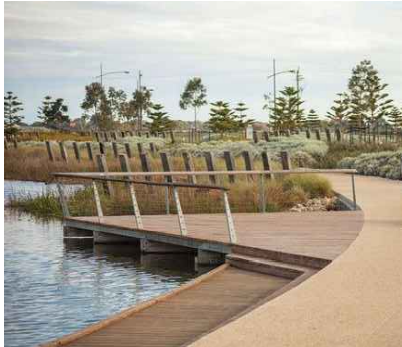
Deck Platform Overlooking Pond
