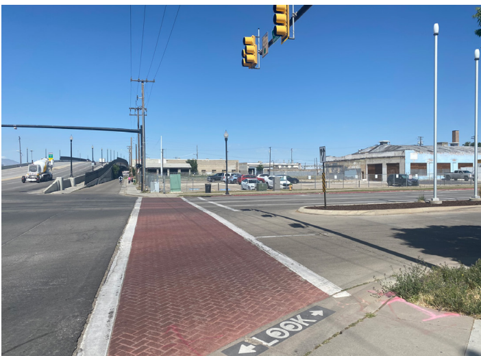
1 View of 500 West and 400 South looking west toward the Blue Warehouse.
