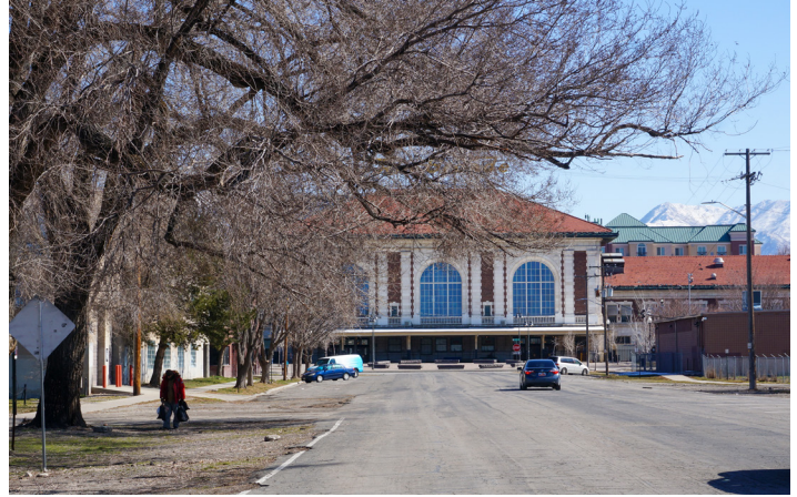
4 View of the Rio Grande Depot looking east from 300 South.
