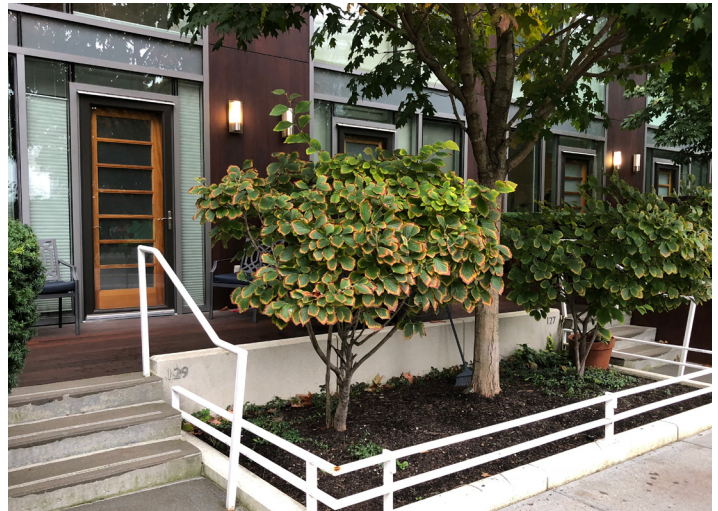
Figure 5.5: Elevated stoops create a semi private space for an intimate social setting.
