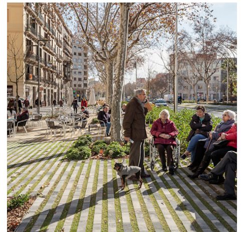
Figure 3.25: Permeable pavers can help with stormwater infiltration and reduction of urban heat island.
