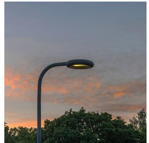
Figure 3.27: Exterior street lights that adhere to dark sky standards help mitigate light pollution and disruption of circadian rhythms.
