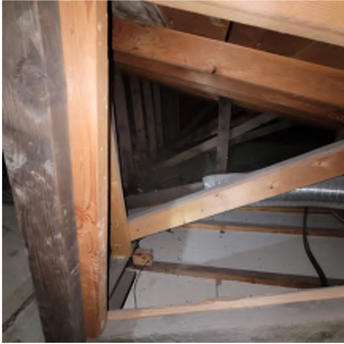
Rear shed roof addition structure
