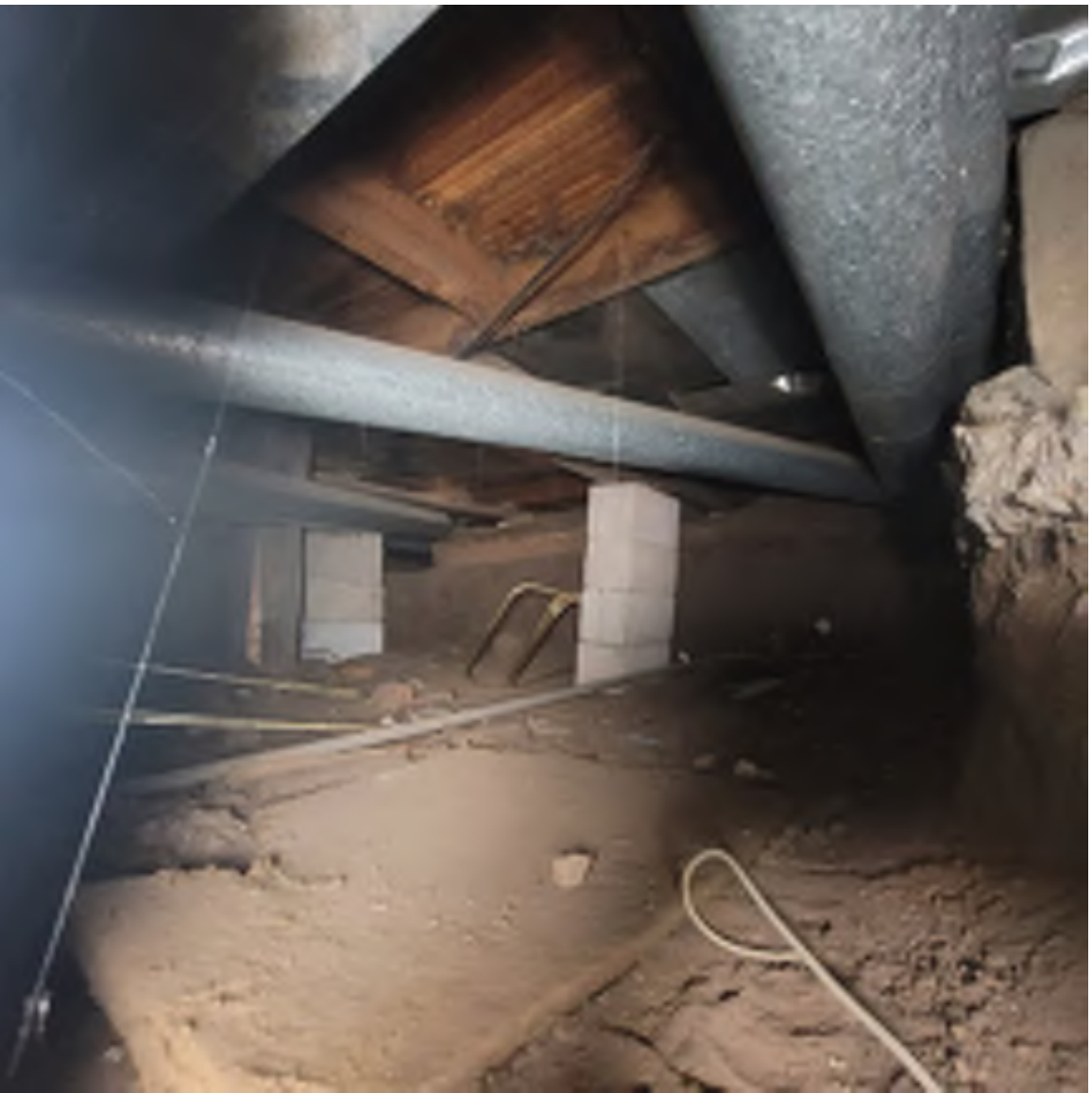
Showing continuous floor for original historic L-shape building form
