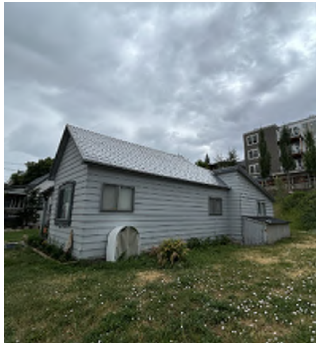
North concrete grade beam perimeter band
