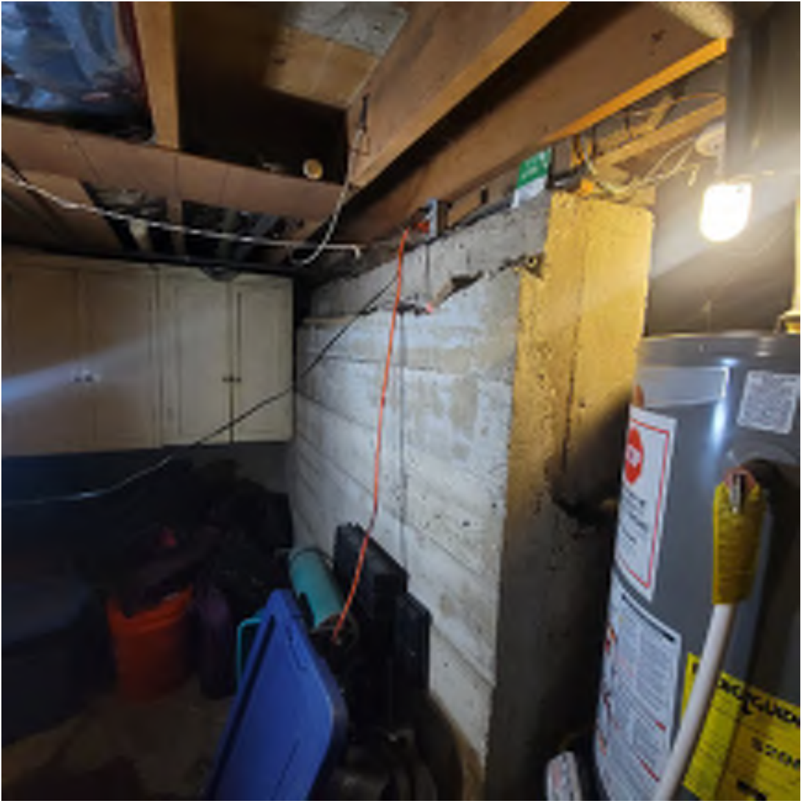
Floor Under Rear Addition of House. Rear addition has new structural members inconsistent with historic L shape structural members
