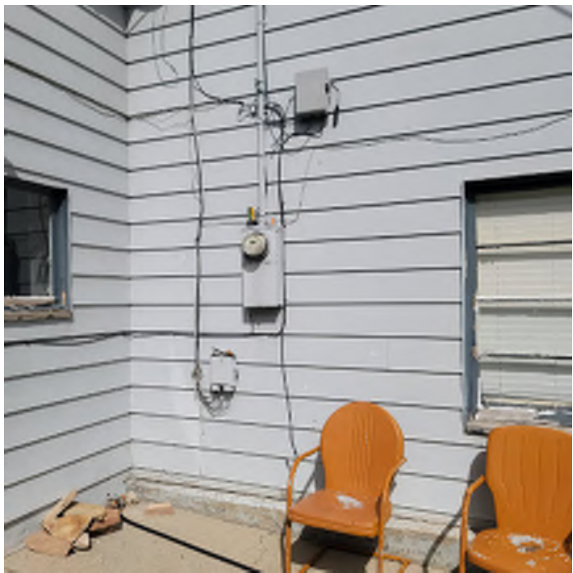
Extent of south concrete grade beam perimeter band
