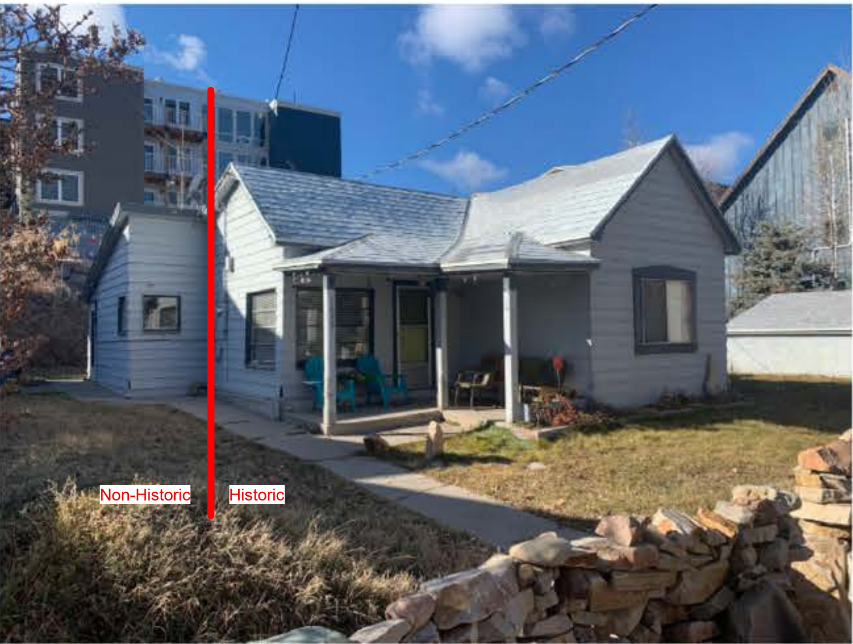
View of Non-Historic Front Porch
