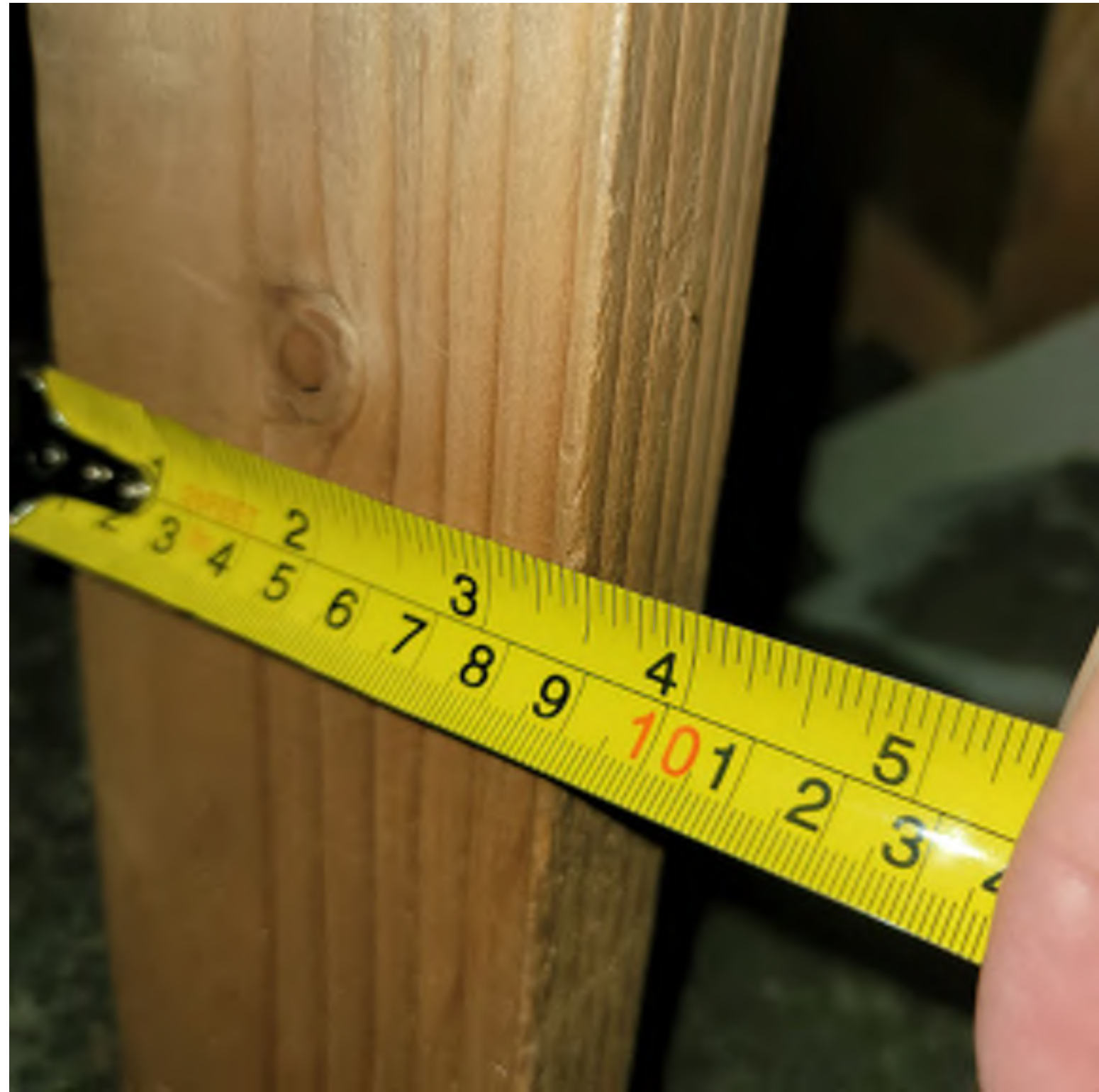
Measurement of an upright in the rear shed roof addition. Showing width and depth of 3 1/2" x 1 1/2" which is modern lumber dimensioning
