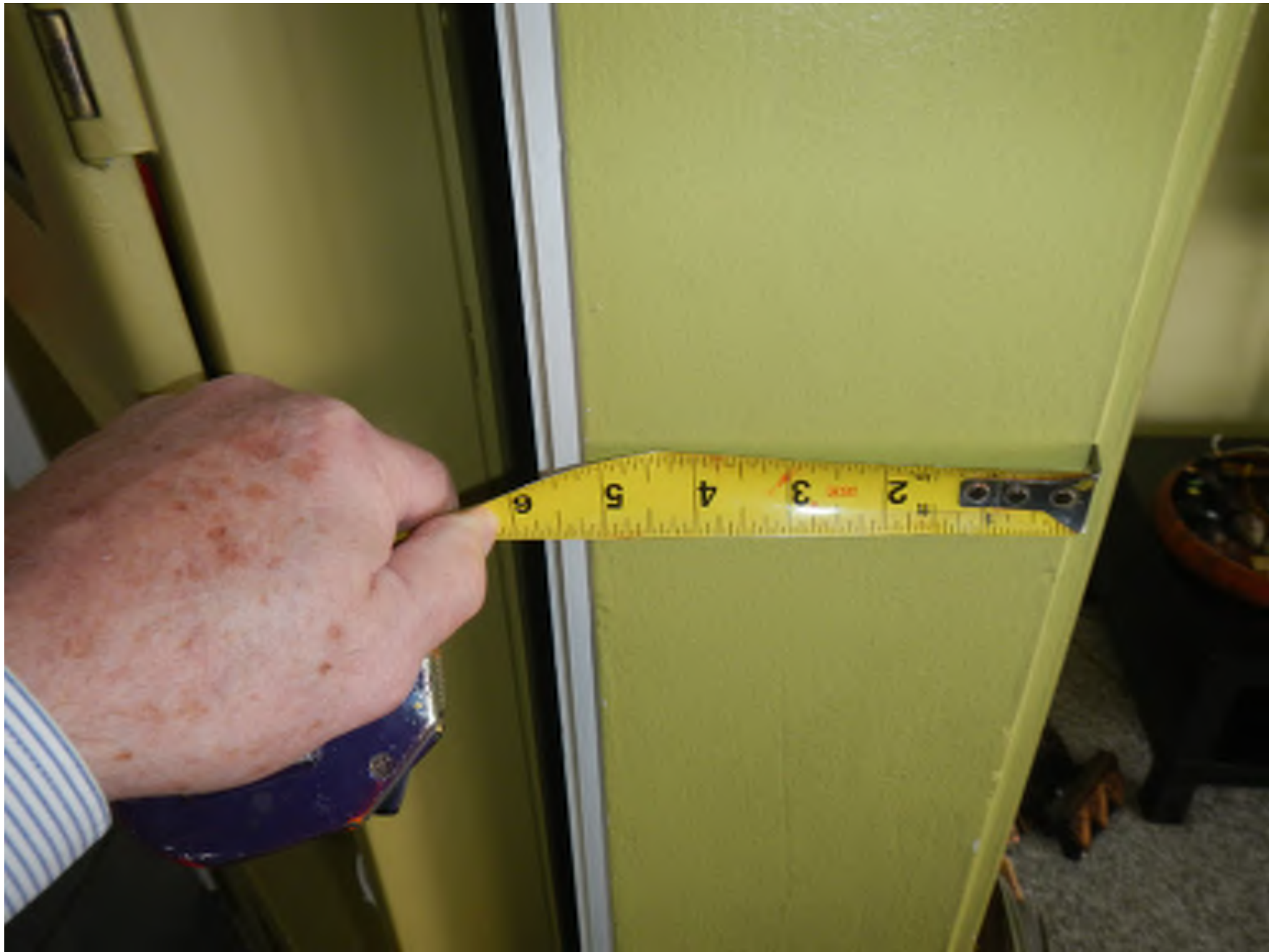
Measurement of original 1904 rear exterior wall between original 1904 L-shape structure and rear addition. Now interior wall
