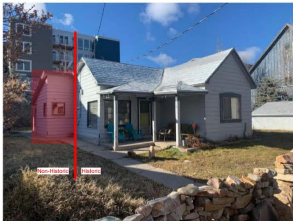
View of Non-Historic Front Porch
