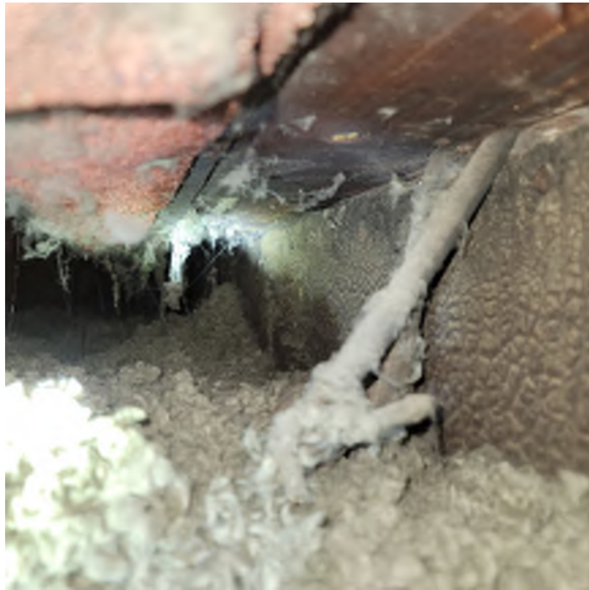
~1904 roof soffit layers
