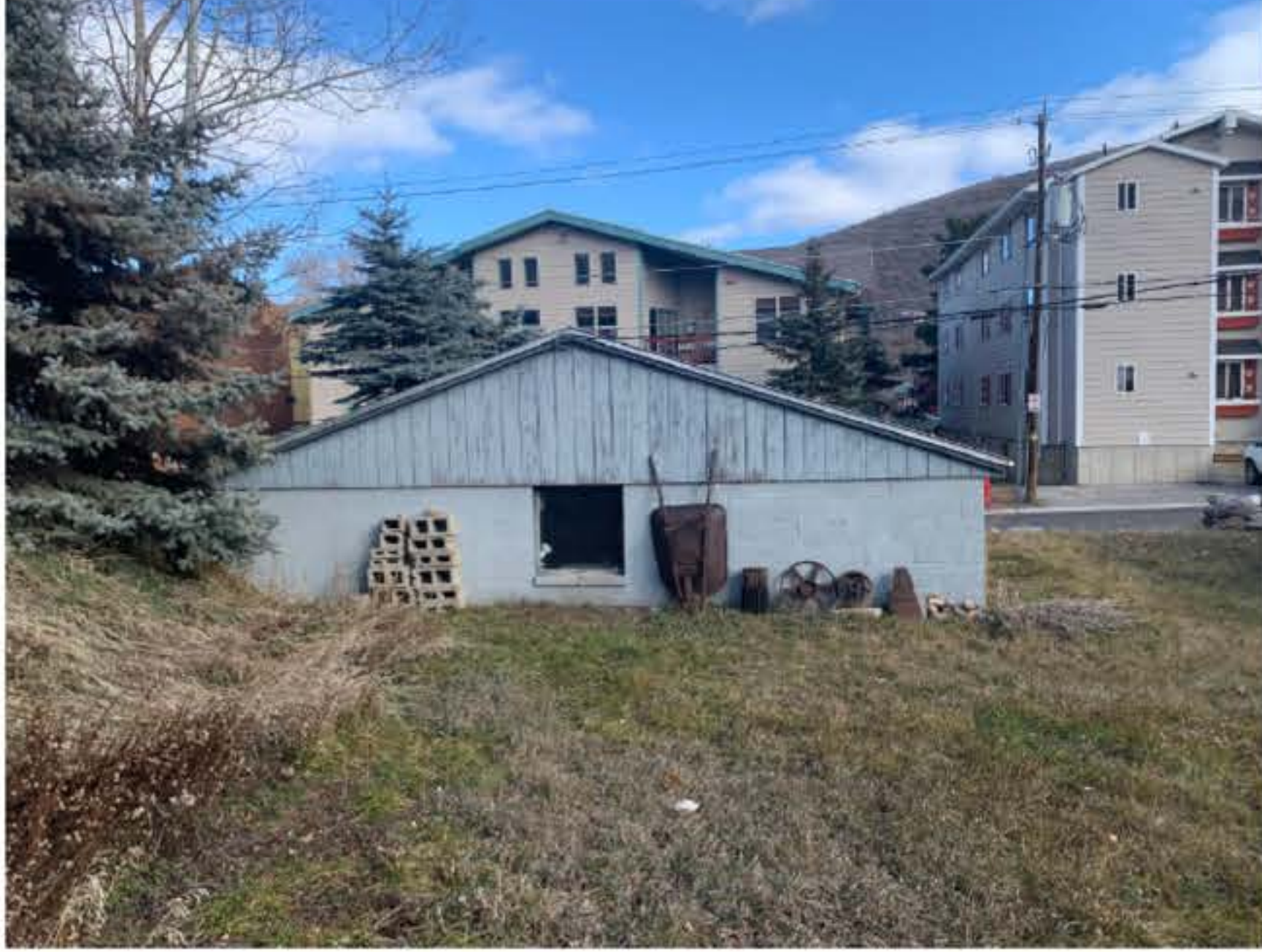
Non-Historic Garage @ Rear
