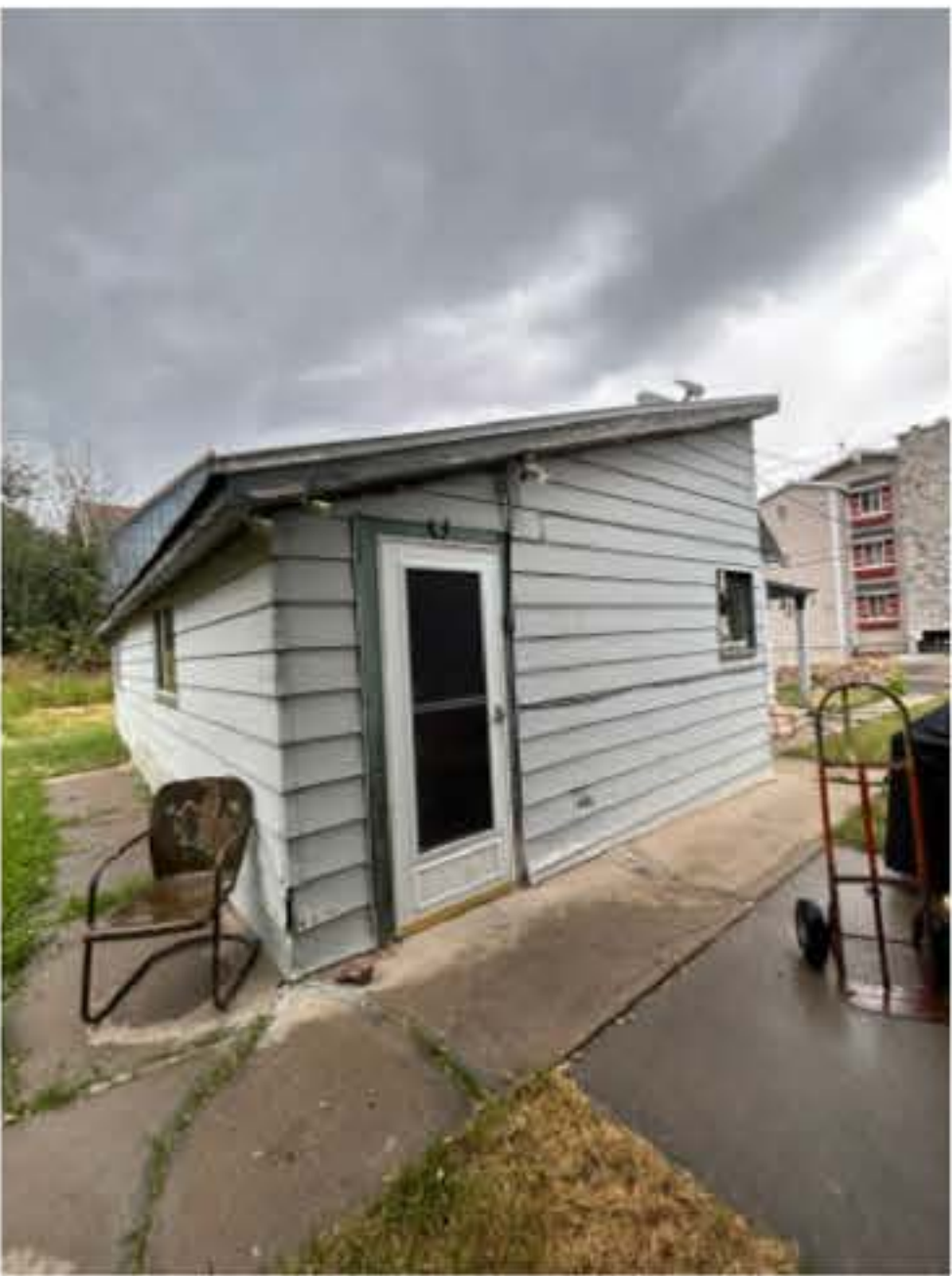
Non-Historic Addition @ Rear
