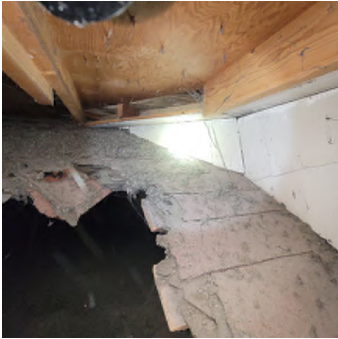
~1904 roof joins with ~1949-1952 rear wall addition
