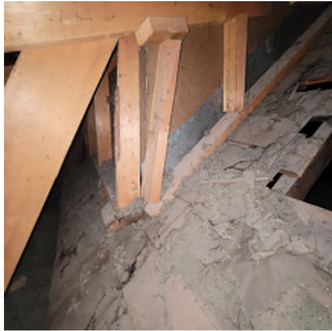
North corner where rear shed roof addition joins with ~1904 roof
