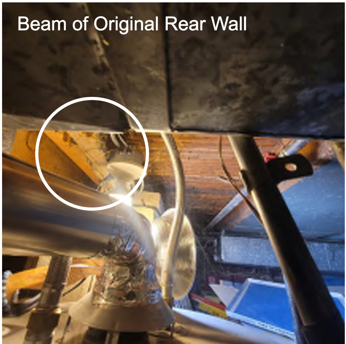
Assumed historic wood timber grade beam visible under house at location of original rear building extents
