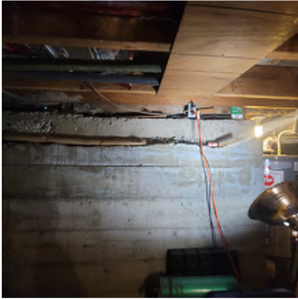
Floor Under Rear Addition of House. Rear addition has new structural members inconsistent with historic L shape structural members
