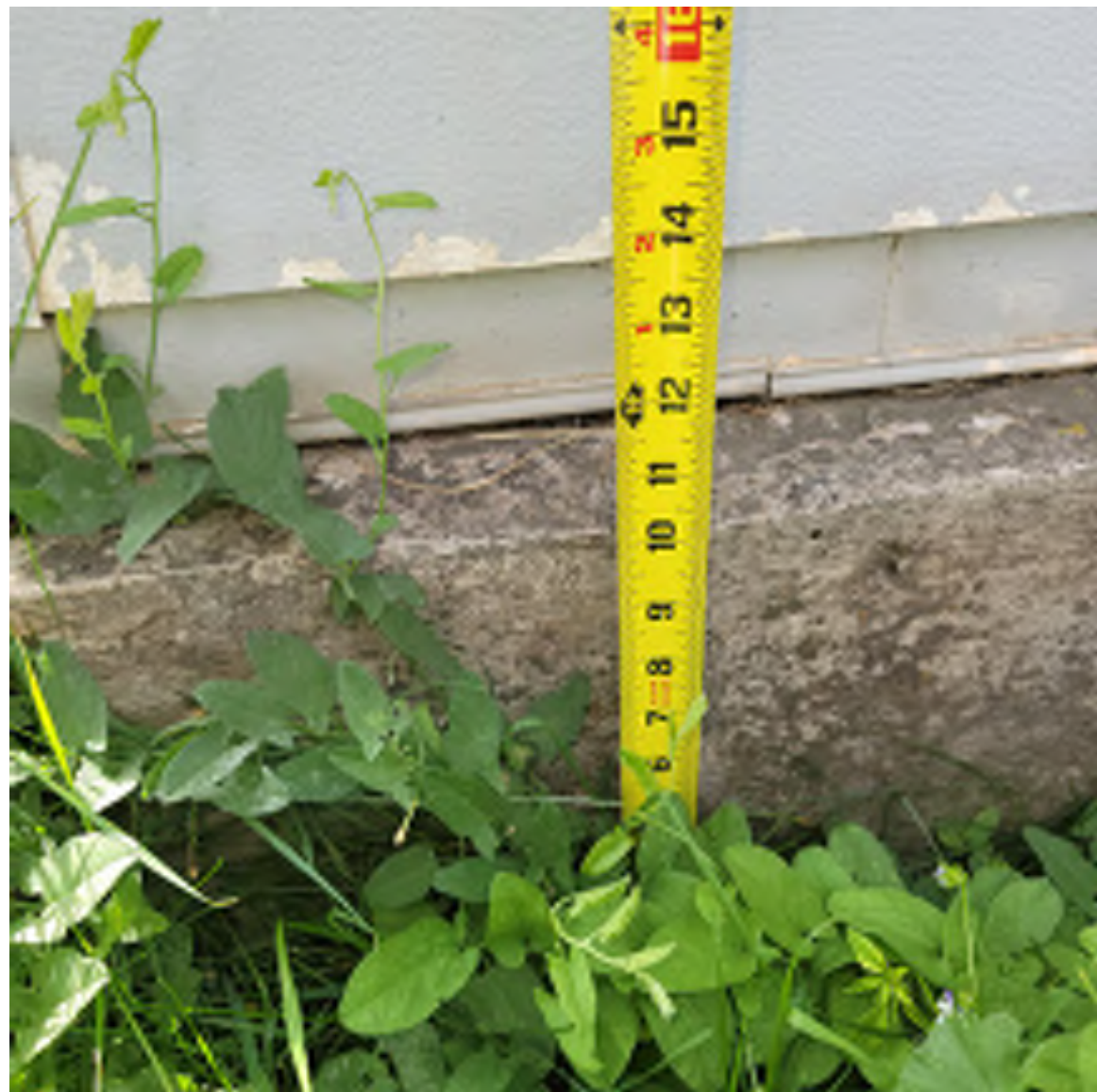
North concrete grade beam perimeter band measurement
