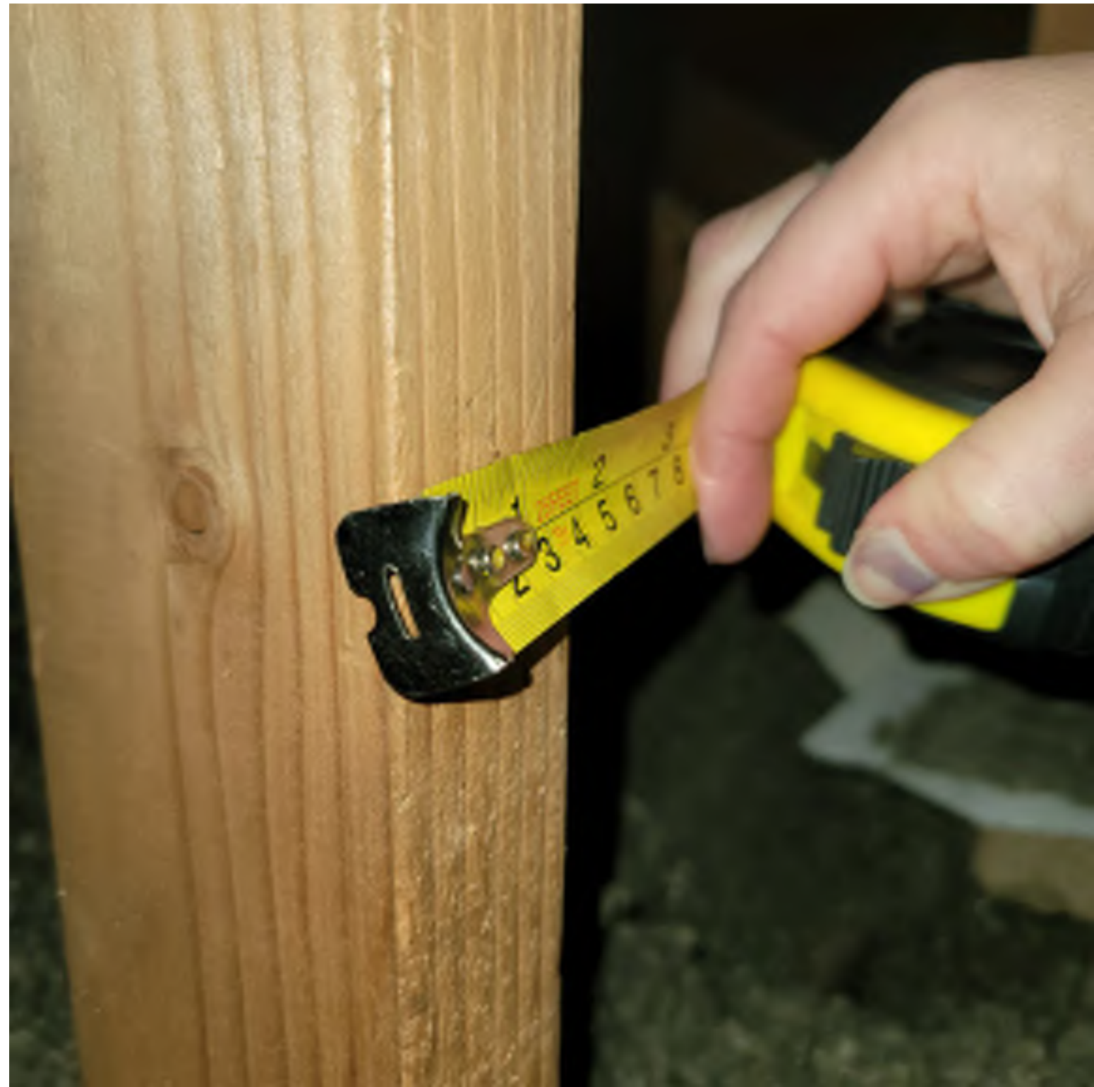
Measurement of an upright in the rear shed roof addition. Showing width and depth of 3 1/2" x 1 1/2" which is modern lumber dimensioning
