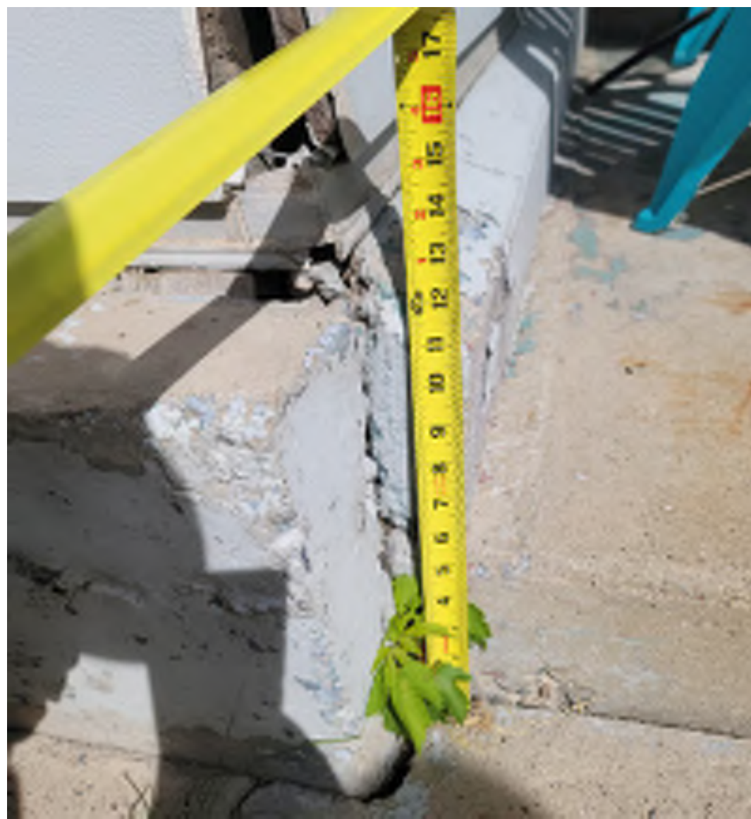
Measurement of southeast concrete grade beam perimeter band
