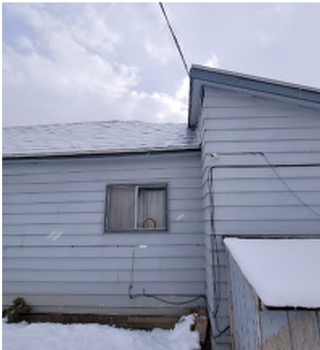
North concrete grade beam perimeter band
