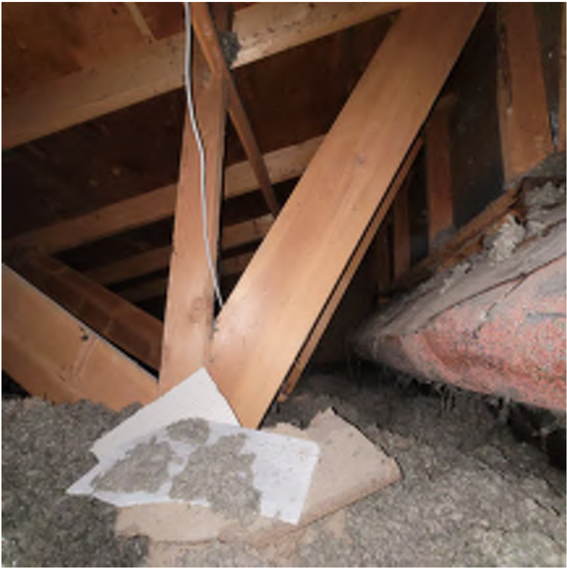
Rear shed roof addition joining with ~1904 roof
