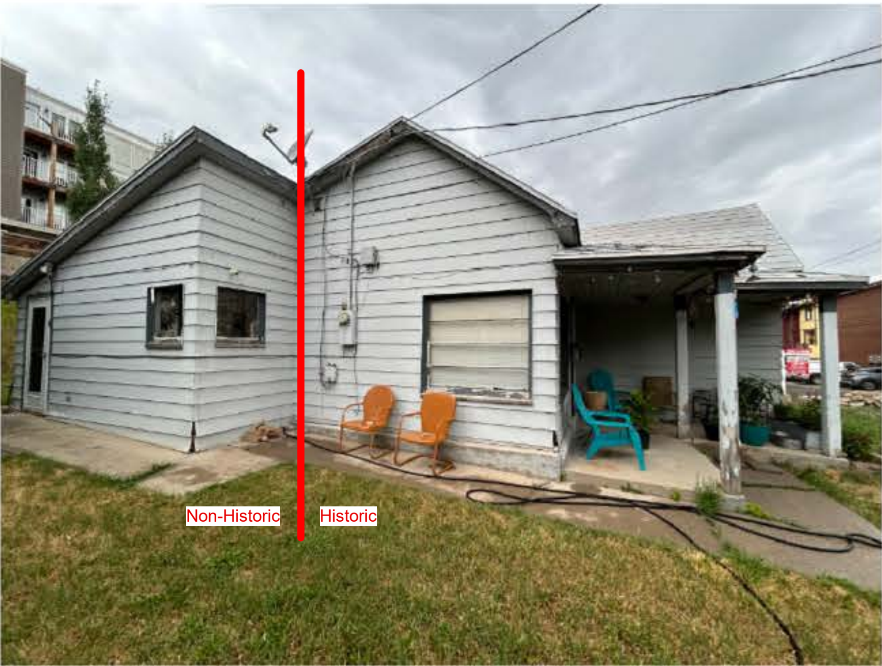
South View of Historic House and Non-Historic Addition
