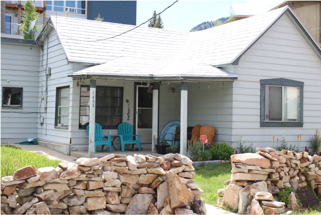
Photo 1: 1455 Woodside Avenue. Southeast oblique. 2020
