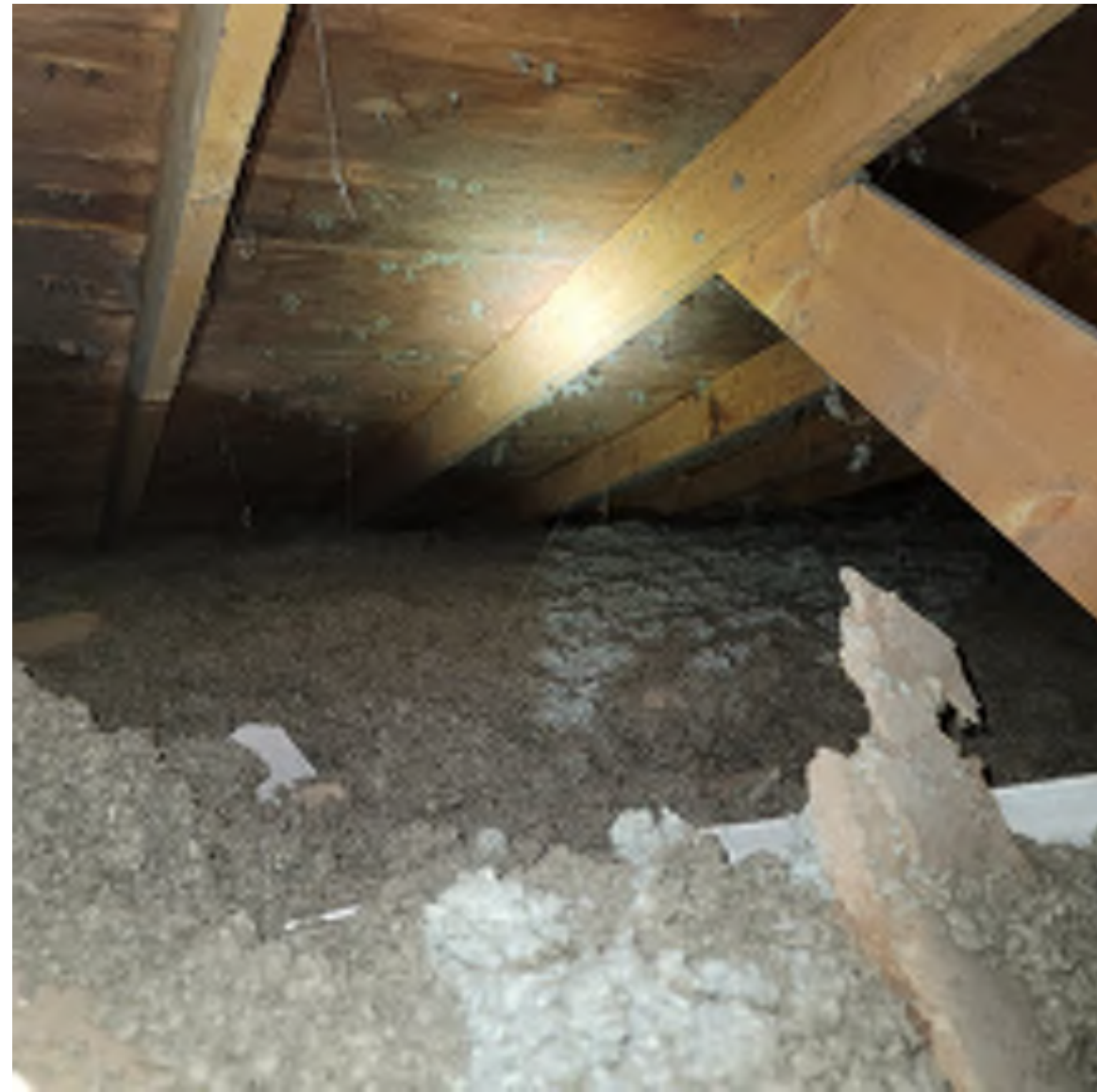
Rear shed roof addition
