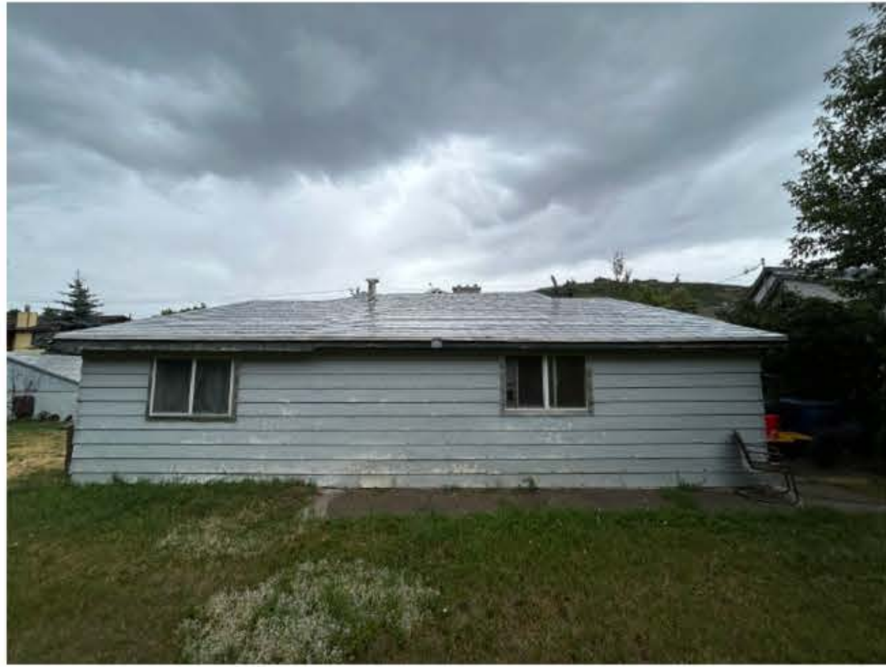
West View of Non-Historic Addition @ Rear
