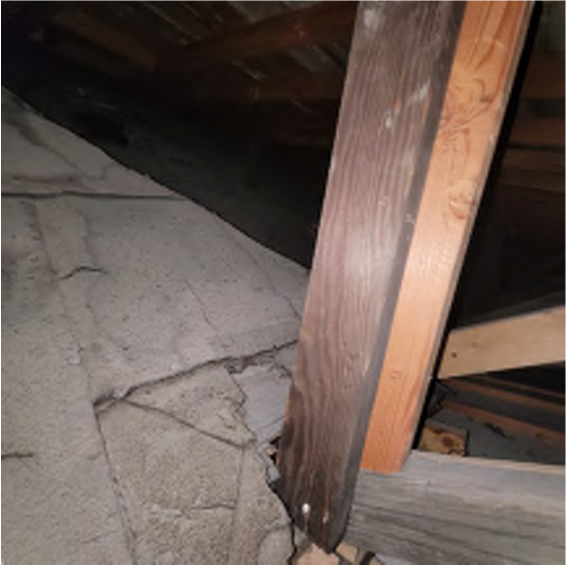
Rear shed roof addition meets ~1904 roof
