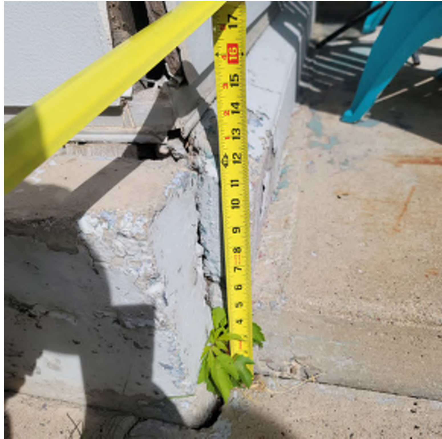
Measurement of concrete grade beam perimeter band (southeast)
