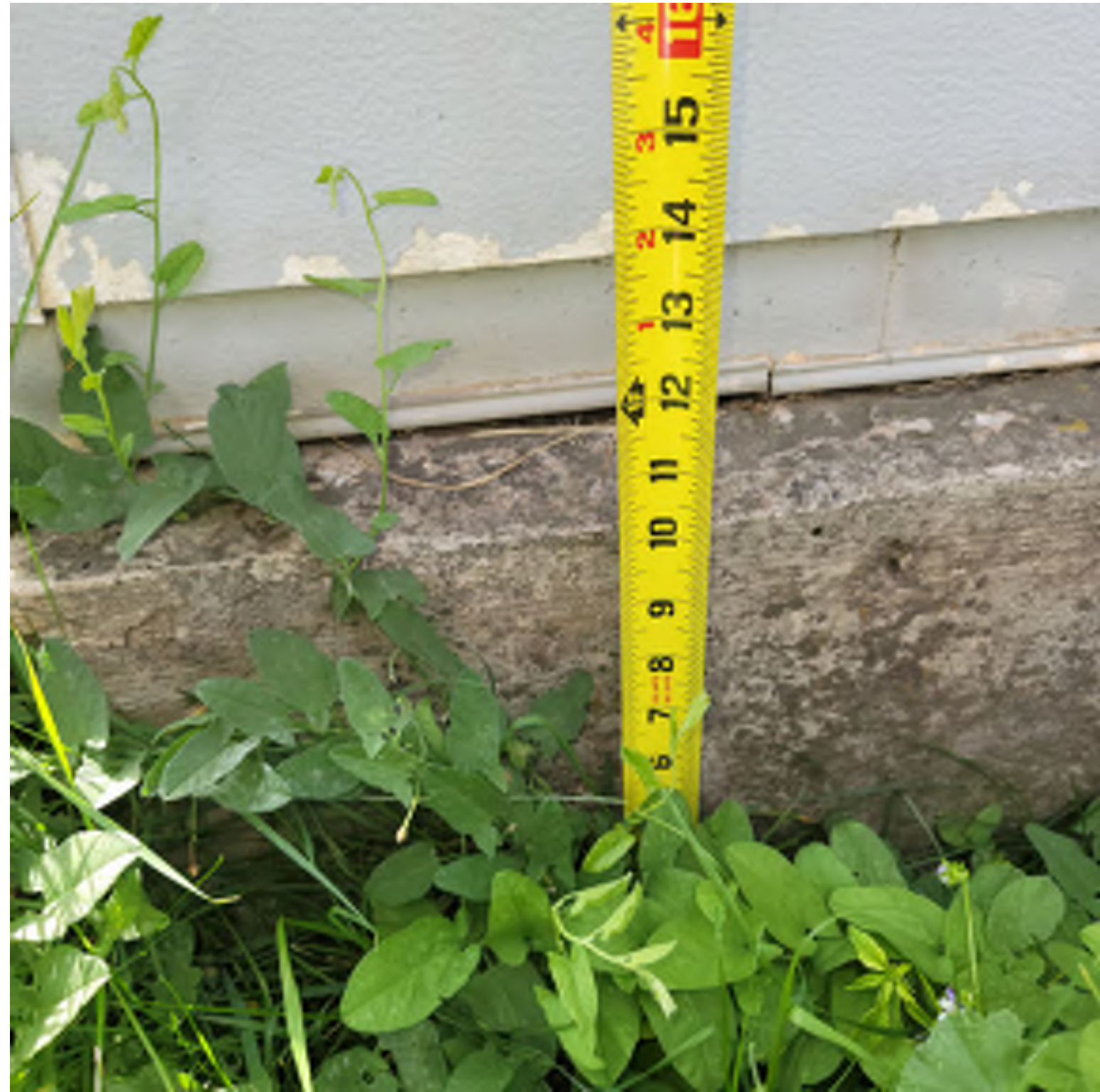
Measurement of concrete grade beam perimeter band (north)
