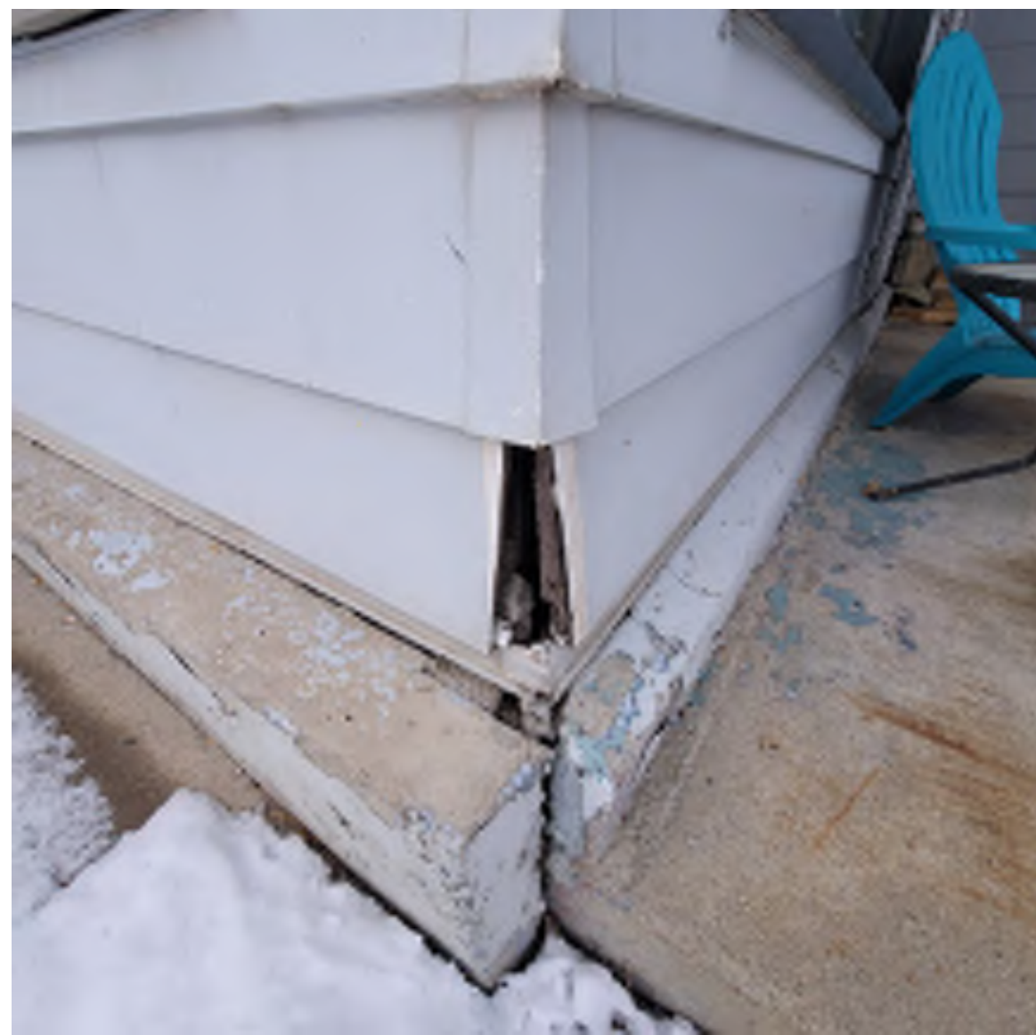
Southeast corner of concrete grade beam perimeter band
