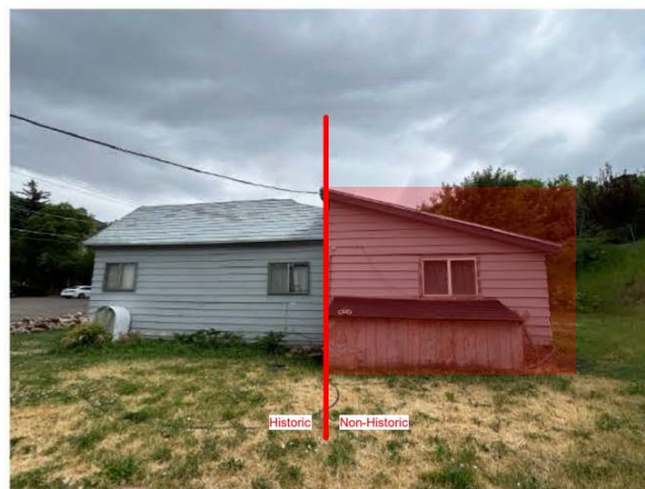
North View of Historic House and Non-Historic Addition
