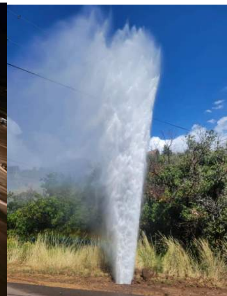
St. Moritz Water line break – 9/15/24
