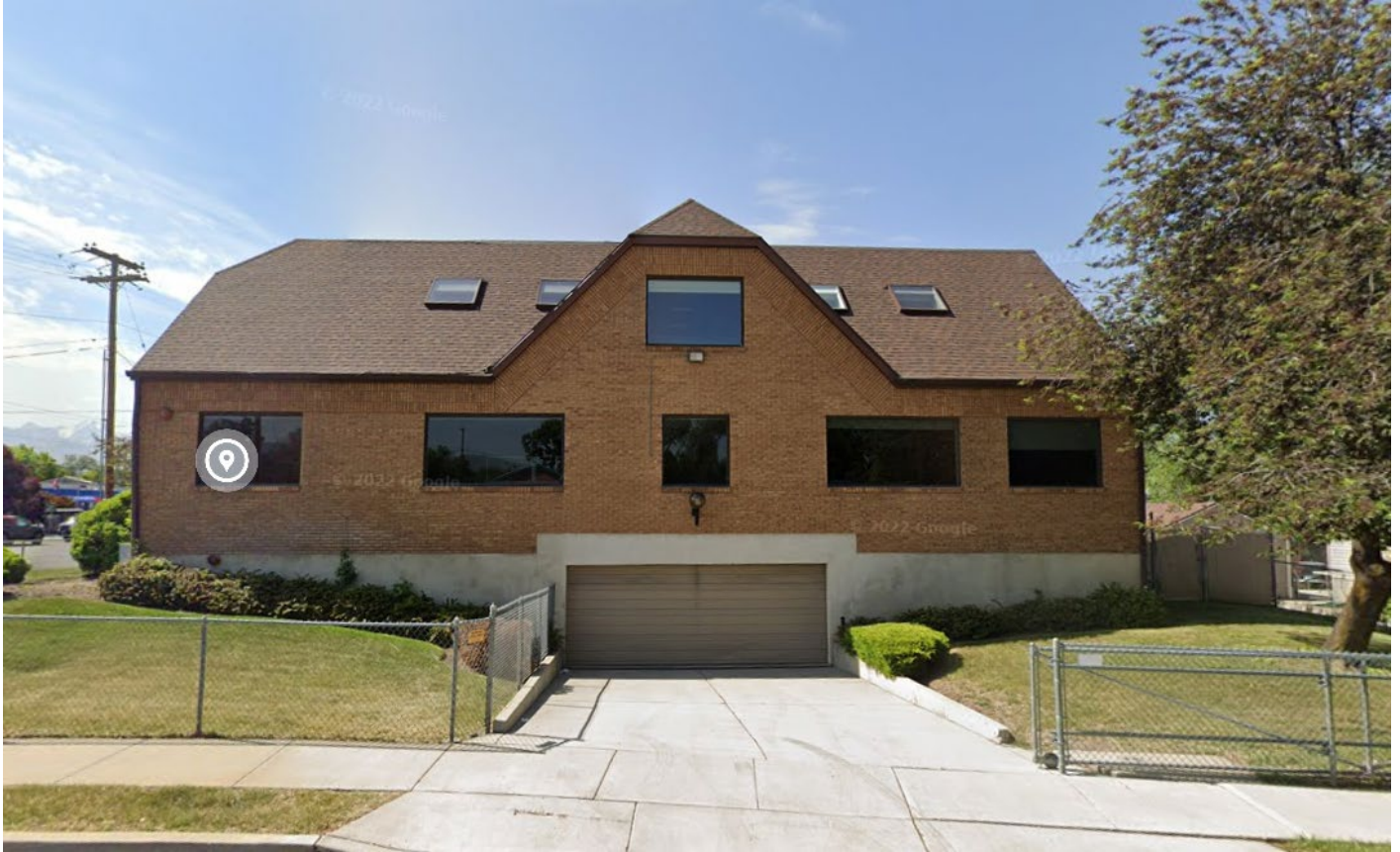
Figure 2: Existing Condition South Facing (3200 S)
