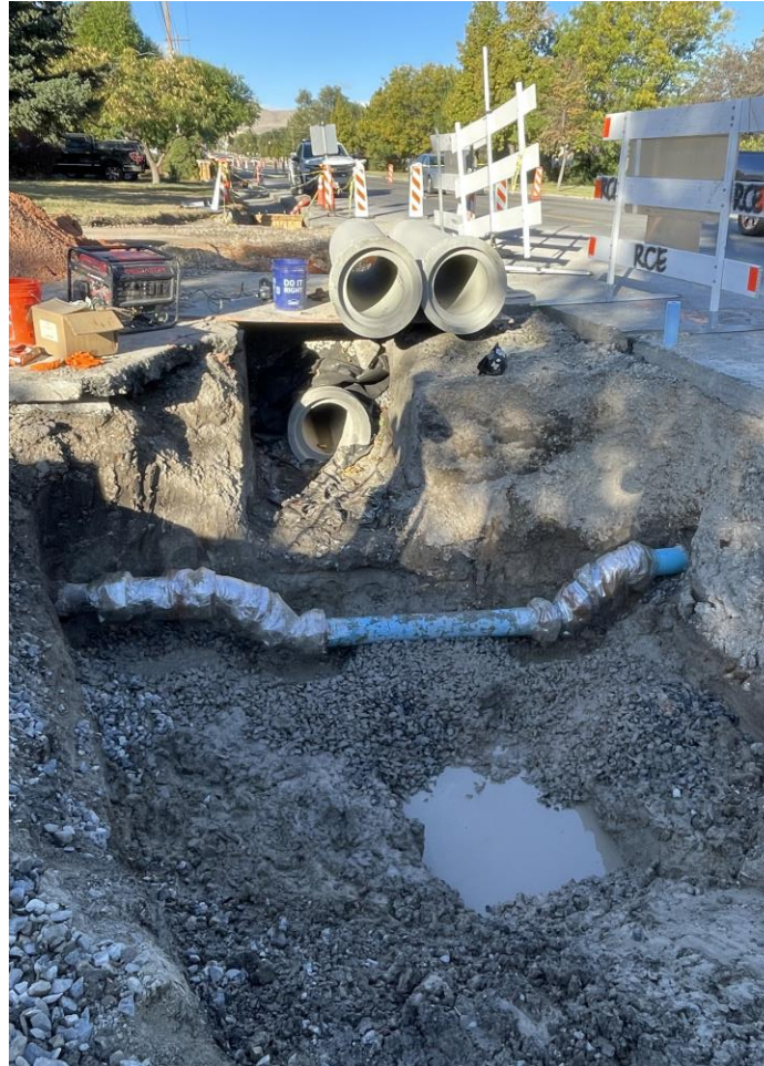
6" water main loop for storm drain conflict
