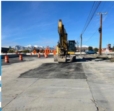
Temporary asphalt patch
