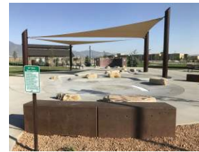
Integral Color Concrete Seat Wall
