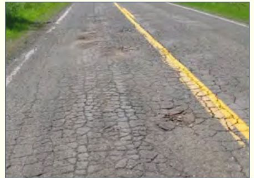
Alligator Cracking
