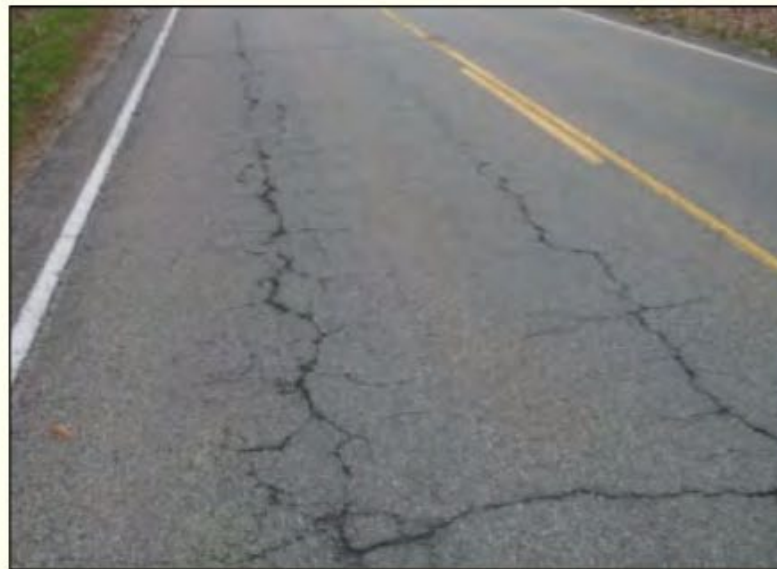
Shear Cracking
