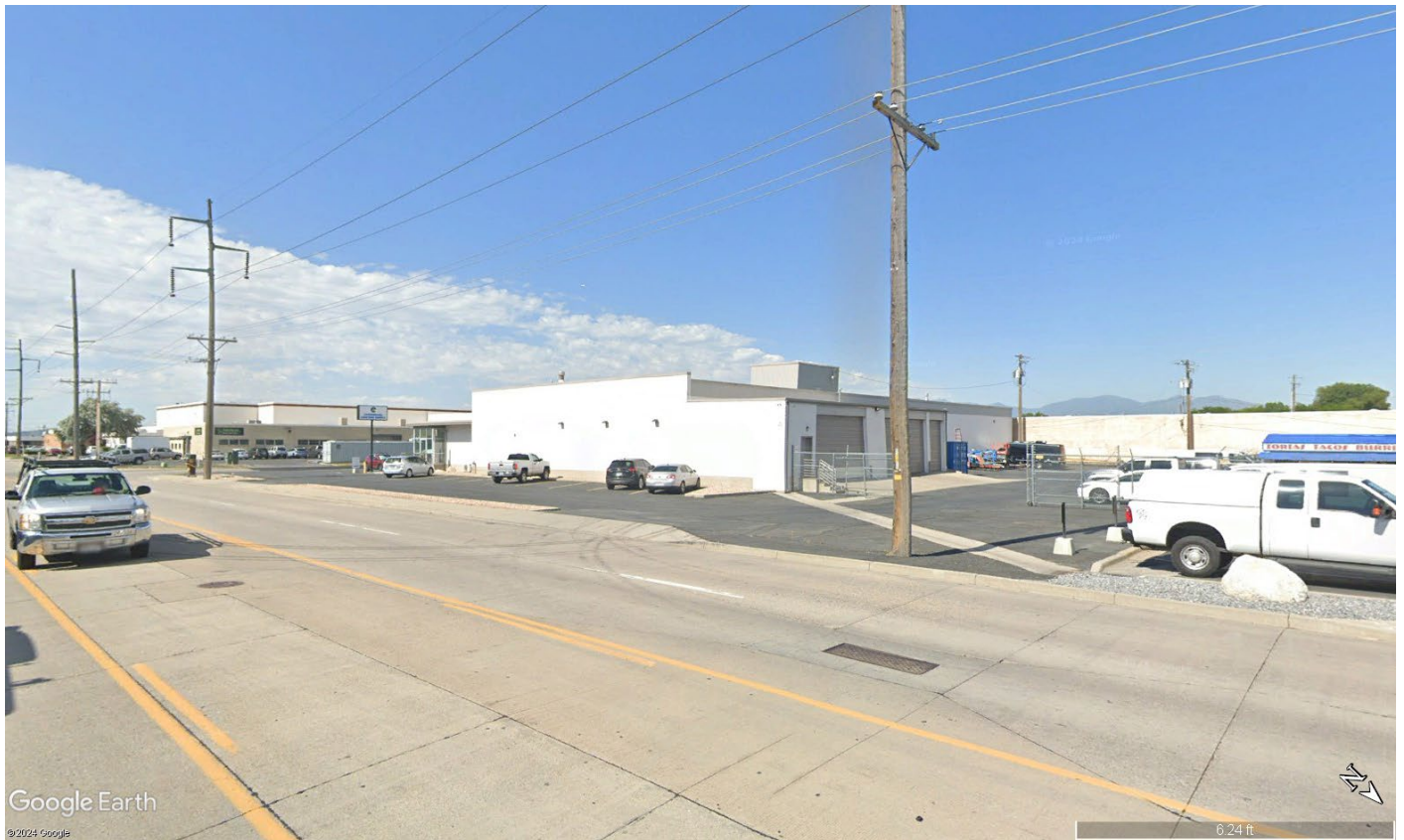
Figure 2: Existing Condition (2264 S 900 W)
