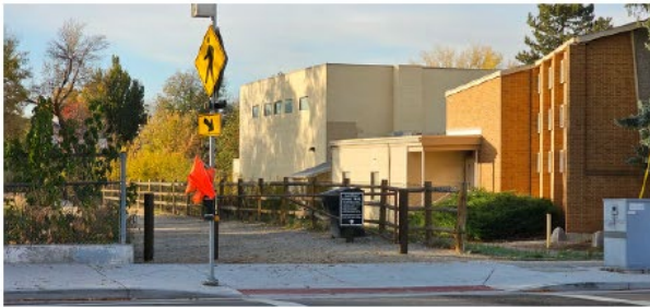
Rapid Flashing Beacon Crossing; Ada Ramps; Vehicle Access Gate; and Boundary Fencing (Post And Rail W/ Chainlink Infill)
