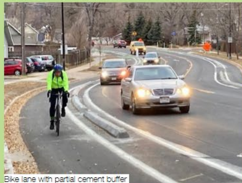
Bike lane with partial cement buffer
