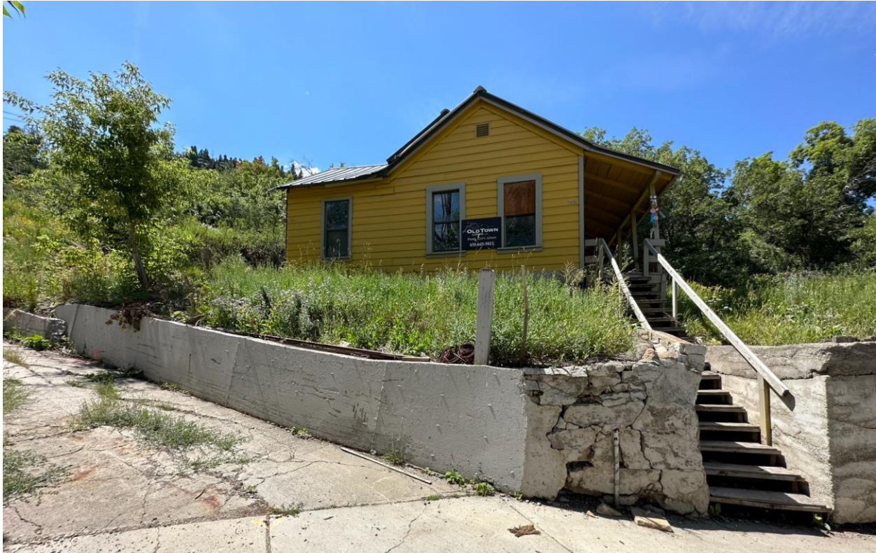
Figure 3: 2023 Photo Submitted by the Applicant, showing the removal of Addition A.
