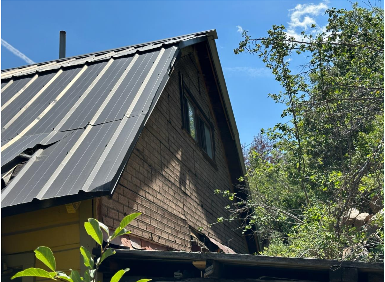
Figure7: Looking easterly, the upper-level Addition F with a faux brick panel façade and gambrel roof; the shed roof of the root cellar, Addition E, is visible at the bottom of the photo.
