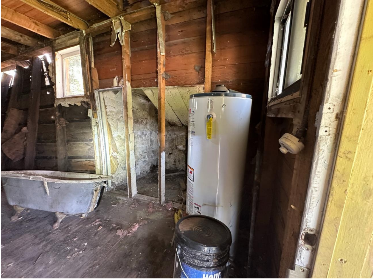
Figure 5: View looking westerly toward Addition E, the root cellar, the area the Applicant proposes constructing a transitional element.
