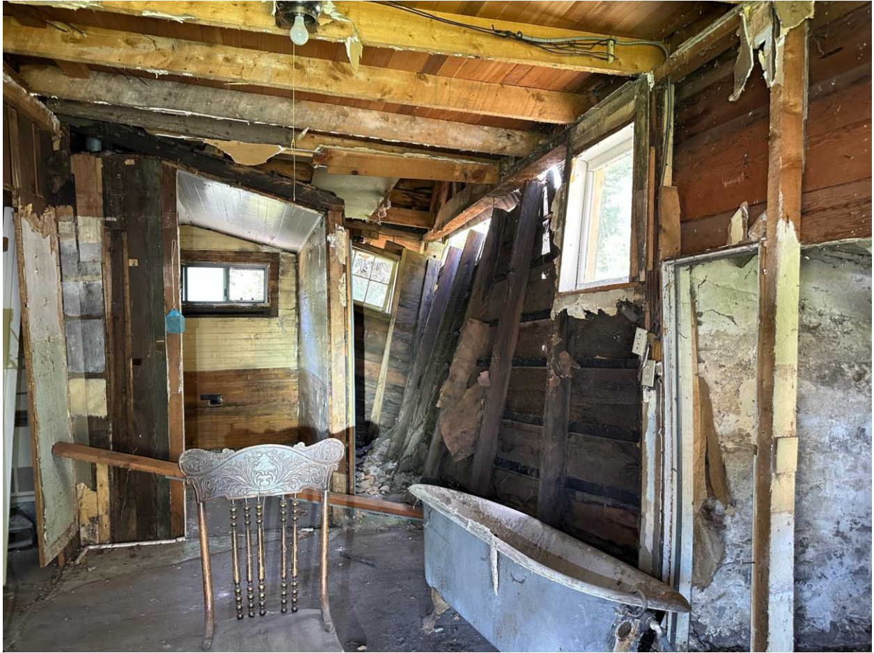
Figure 4: Looking southerly, Additions B and C to the back of the photo; the root cellar, Addition E, the root cellar, can be seen to the right of the photo.
