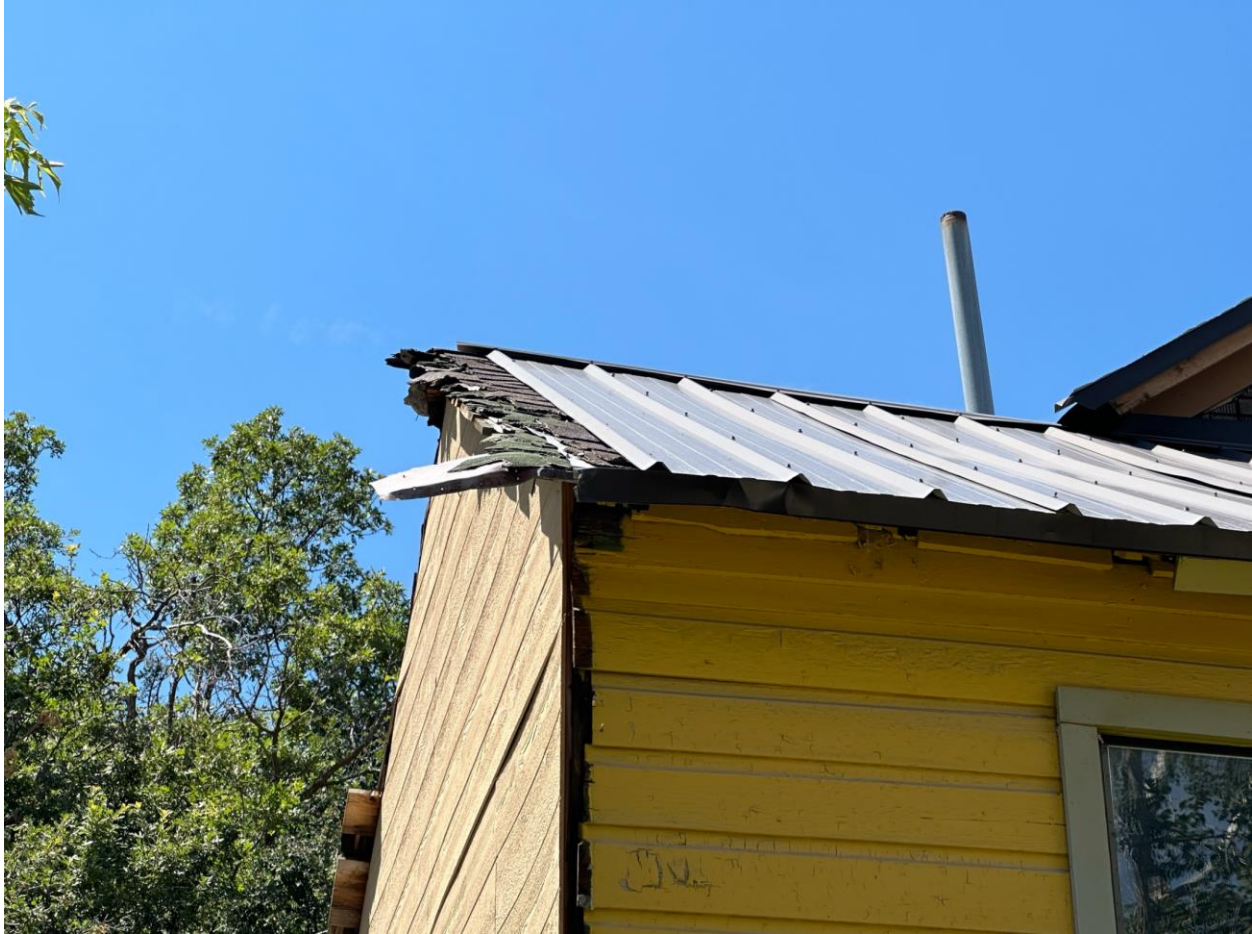
Figure 9: Addition A was removed, and temporary siding installed.
