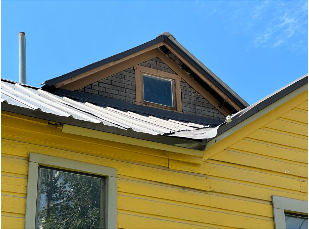
Figure 8: Looking westerly, Addition F, the upper-level addition remains, clad in faux brick panels.
