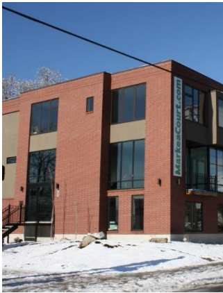
Primary Materials: Bricks
