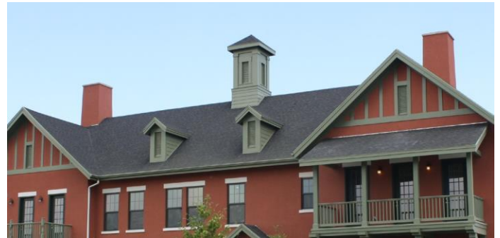
Roof Materials: Asphalt Composite Shingles
