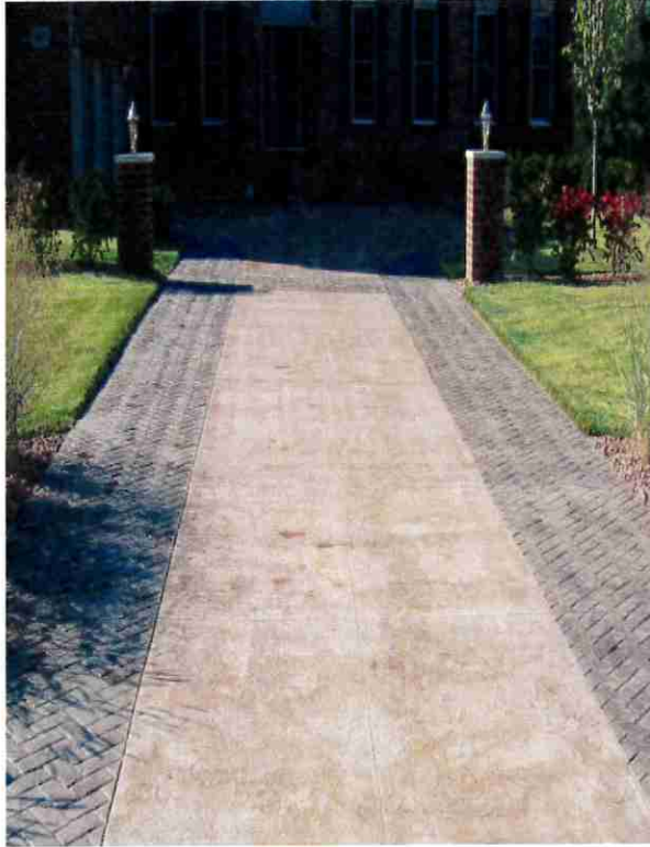
Stamped concrete. Photo courtesy of Todd's Services.
