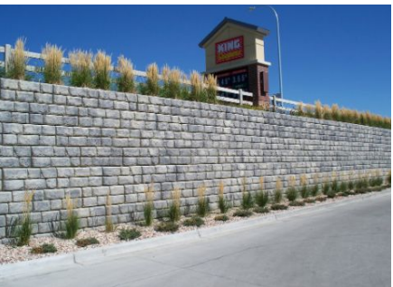
Example of roadway fencing
