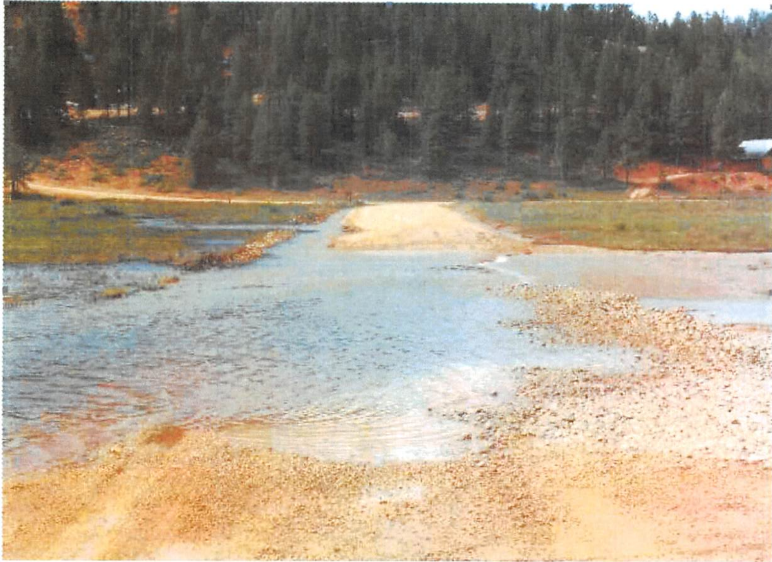
This is a photo taken of flooding across Meadow Lane at the corner of Meadow Lane and Strawberry Point Road. Recently a new culvert was placed along Willis creek raising the road about 2 feet over the creek bed. This helps prevent overflow from the creek directly, but water runoff from the meadow still travels across Meadow Lane. Base leg's property is on the right side of Meadow Lane. The meadow property floods every year.
