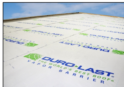
6. Once installation is complete, the Duro-Last Vapor Barrier membrane temporarily protects against inclement weather. If not immediately covered, follow extra steps per 3a and 3b in the instructions above.
