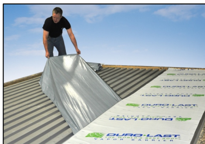
2. Once the membrane is in place, while holding the membrane tight, peel off the silicone release film by pulling diagonally.
