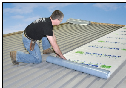
1. Roll out the Duro-Last Vapor Barrier over a clean, dry deck.
