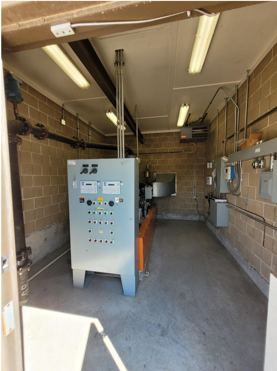
2700 W Lift Station Dual System Controls for AC and DC Application
