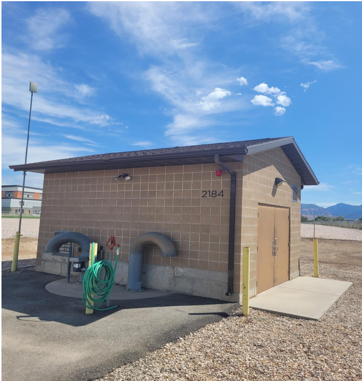
2700 W Lift Station, Showing Wet-Well Half Under Building.
