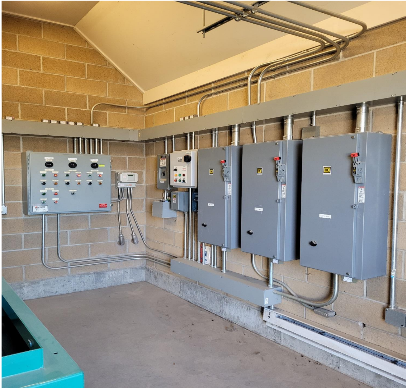
4450 W Lift Station: The three cabinets on the left are the on/off switches for the Pumps.
