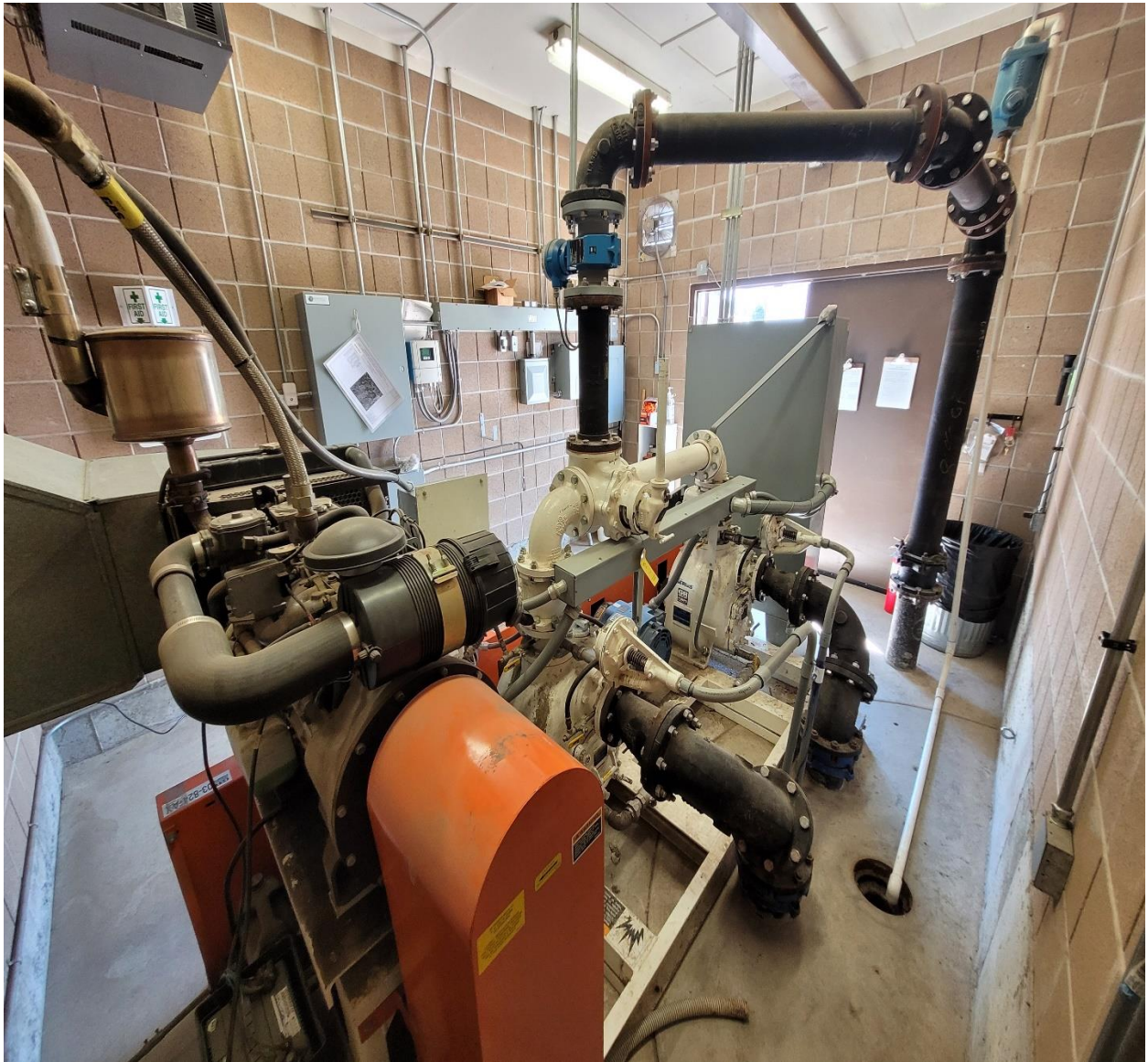
2700 W Lift Station Two Pumps, Back Up Motor, Other Half of Wet-Well
