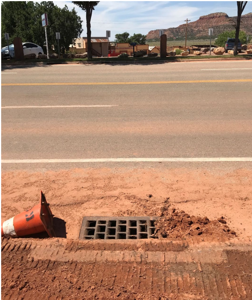
Figure 2-7. Sediment covering the street and sidewalk at 250 West Center Street.
