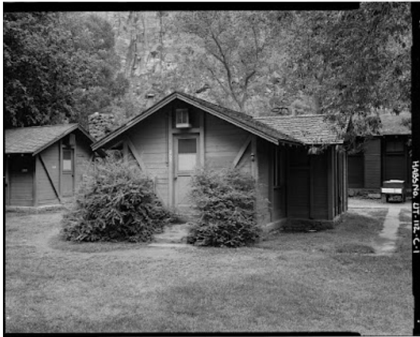
Figure 2. The same, or similar cabins in use at Zion National Park, many years ago
