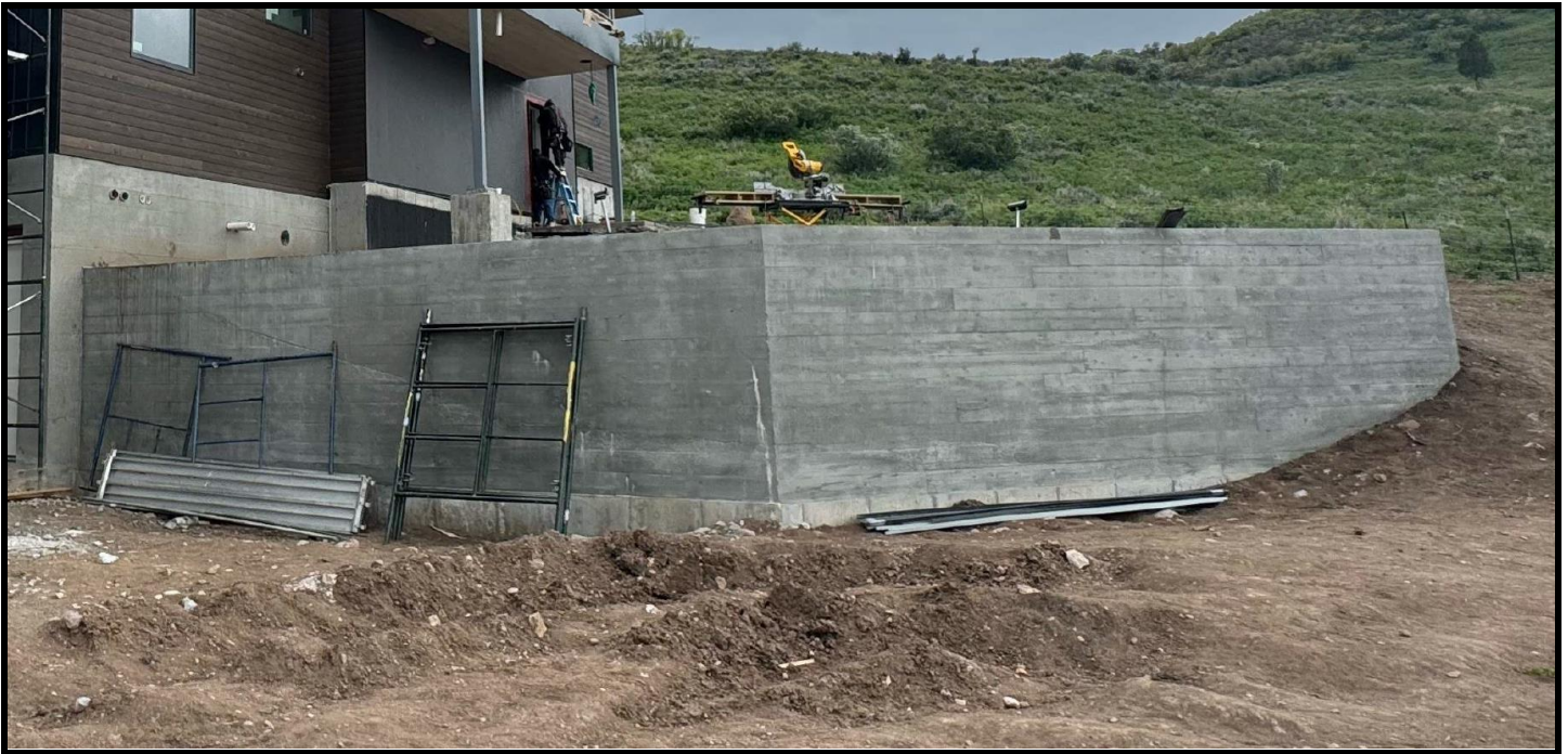
Example Image of Board-Form Concrete Wall
