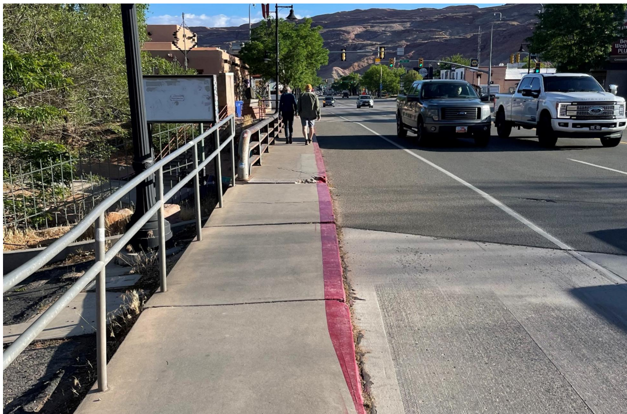
Photograph 24 – Narrow Sidewalk and Low Bridge Rail on Existing Bridge Structure
