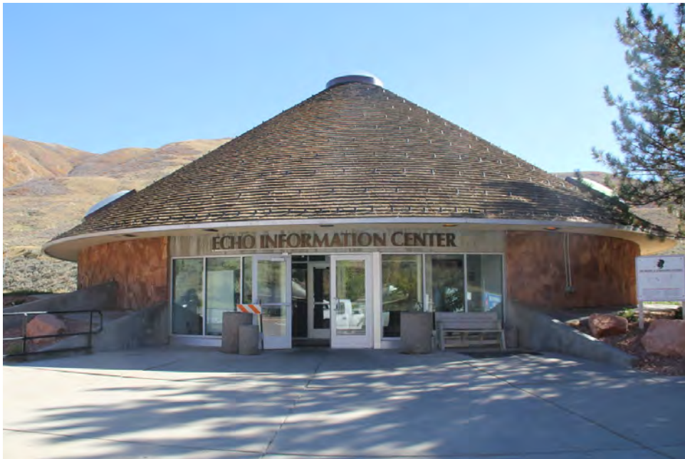
Figure 12. North Interstate 80 Rest Area building; Late 20th Century (Other); ca. 1960.
