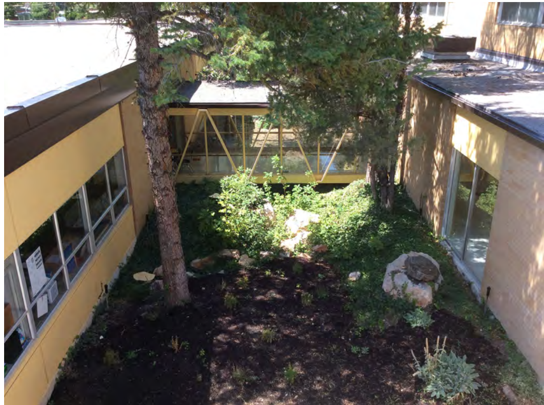
Interior Courtyard and Truss Bridges
