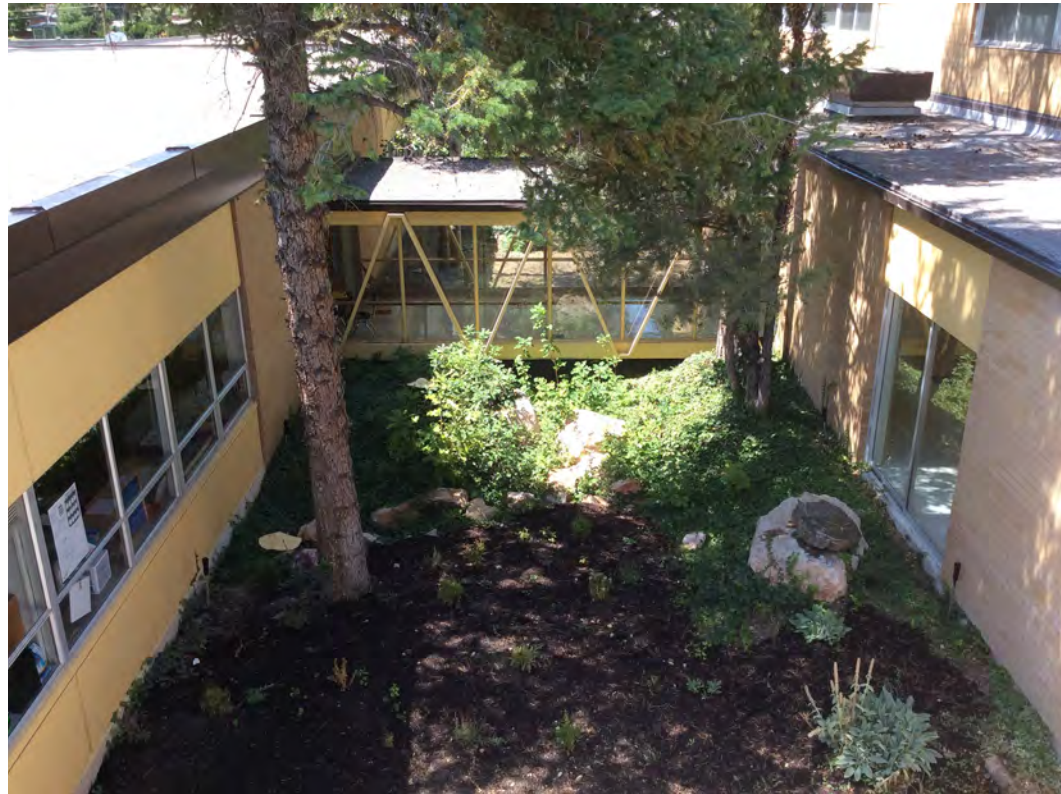
Interior Courtyard and Truss Bridges
