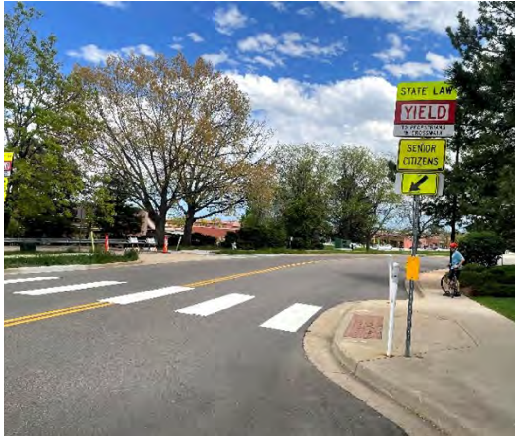
Figure 1: Crossing example with marked crosswalk, signage, ADA curb ramps, and curb extension at marked crosswalk
