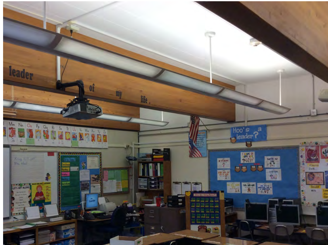
Spring Lane Classroom with Exposed Glulam Beams
