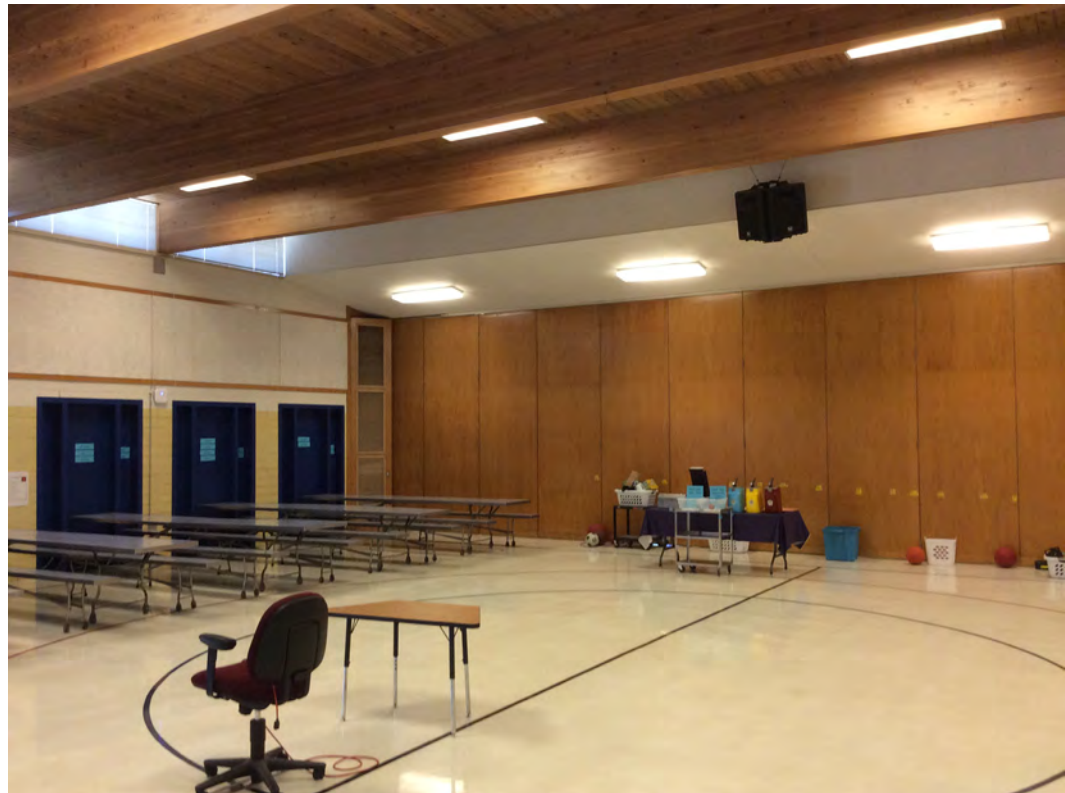
Multi-Purpose Room with Glulam Beams
