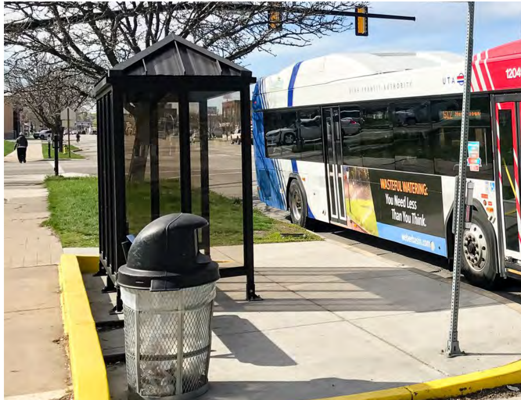
UTA Enhanced Bus Stop Source: UTA
