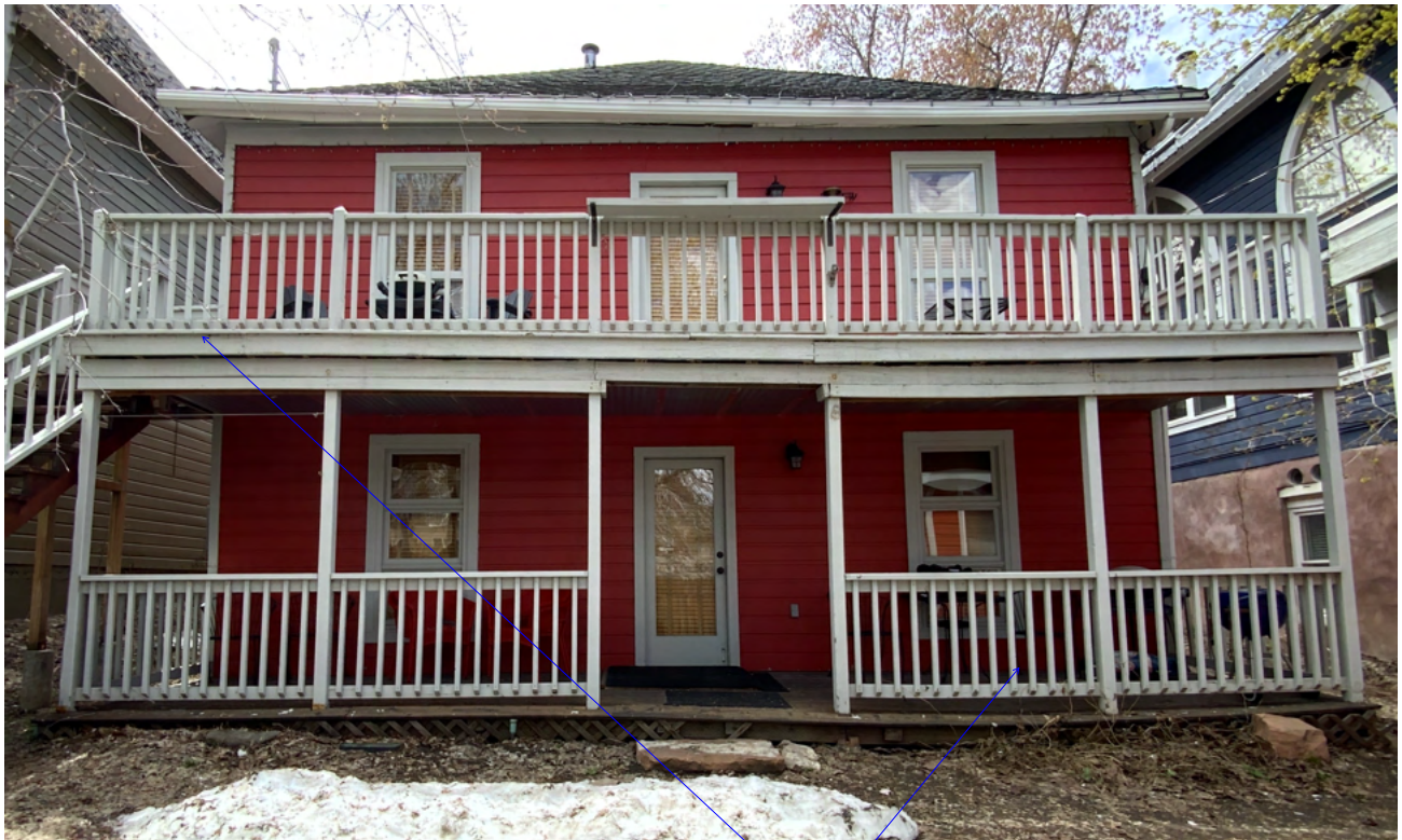
PHOTO 3: BACK ELEVATION SHOW DECK
