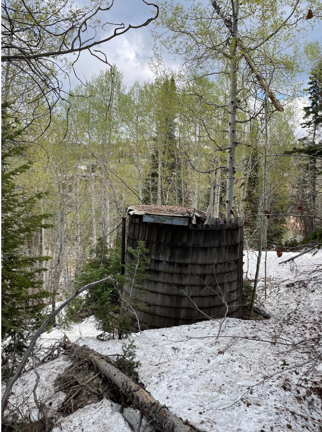
Figure 2: Water Tank E
