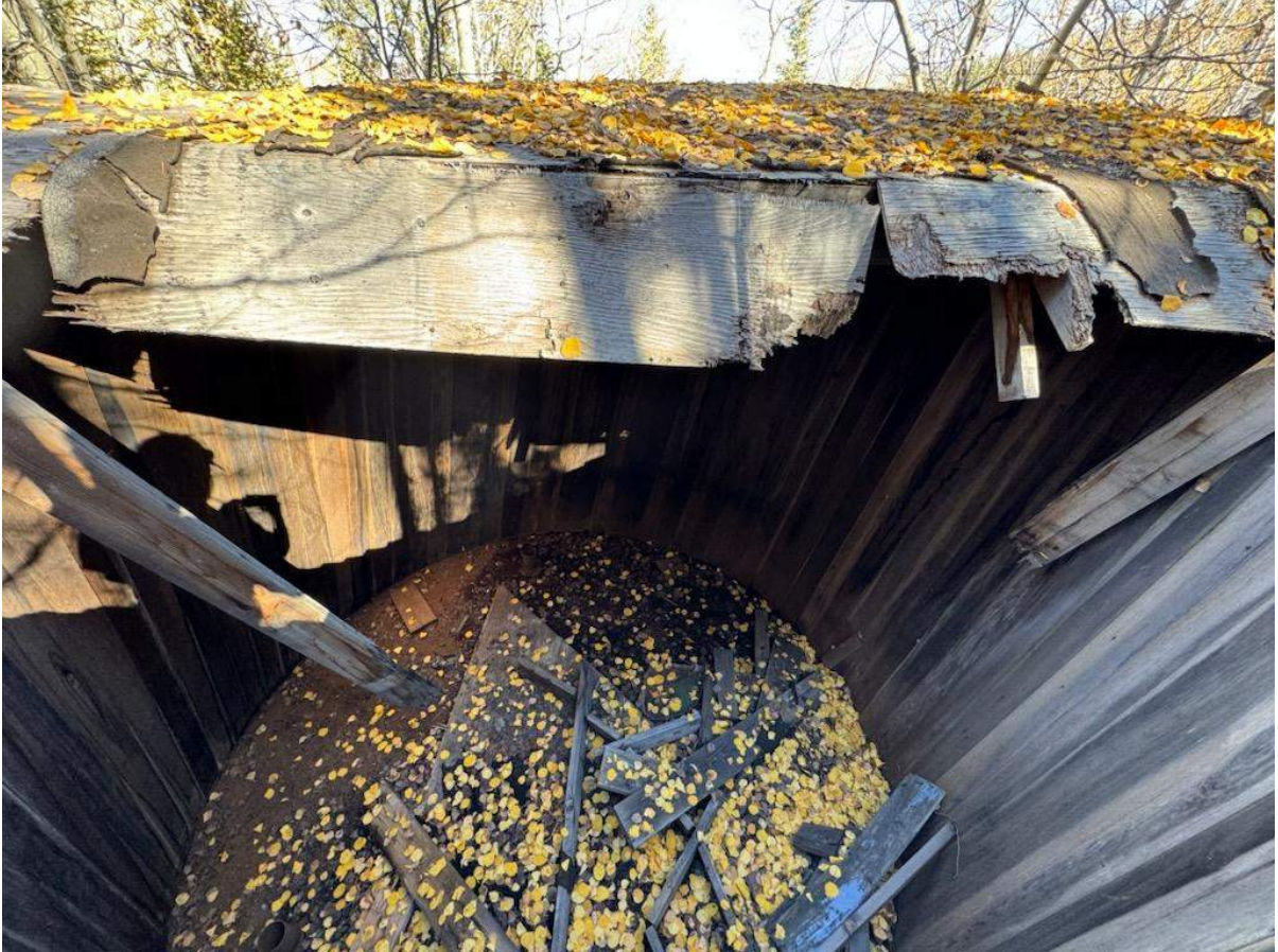
Photo 4—Water tank roof condition
