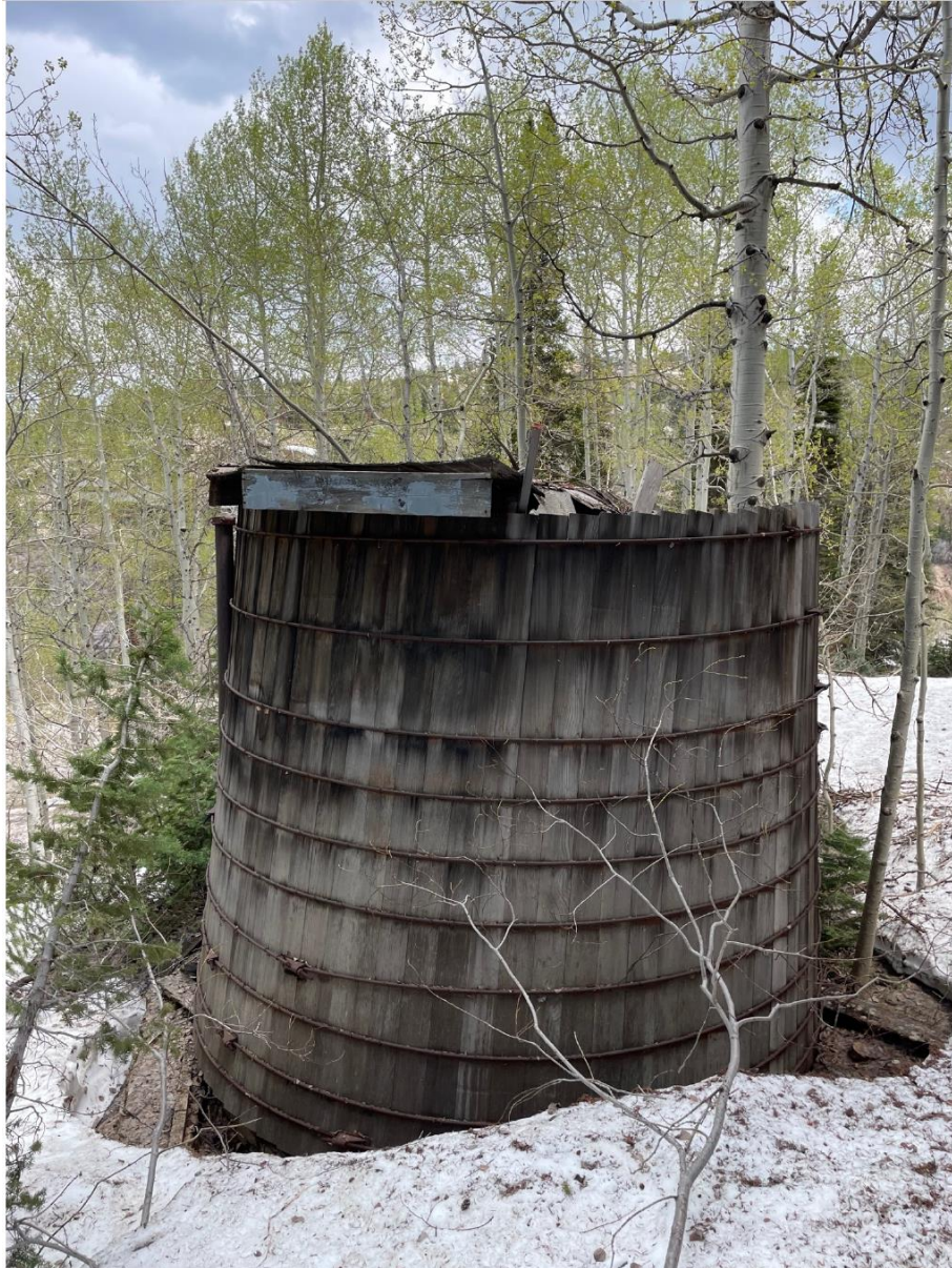
Figure 1: Water Tank E
