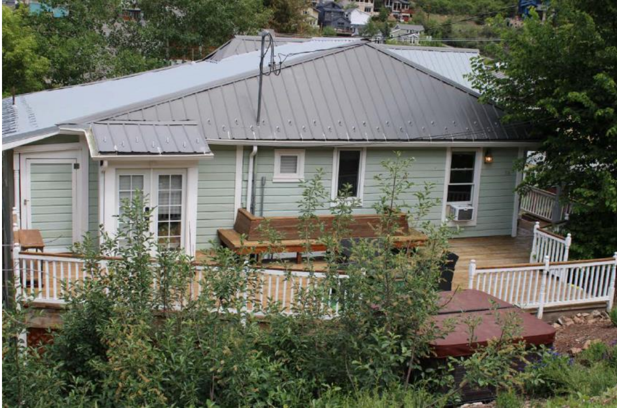
Figure 4: Side facade showing the Historic bay window altered with French doors
