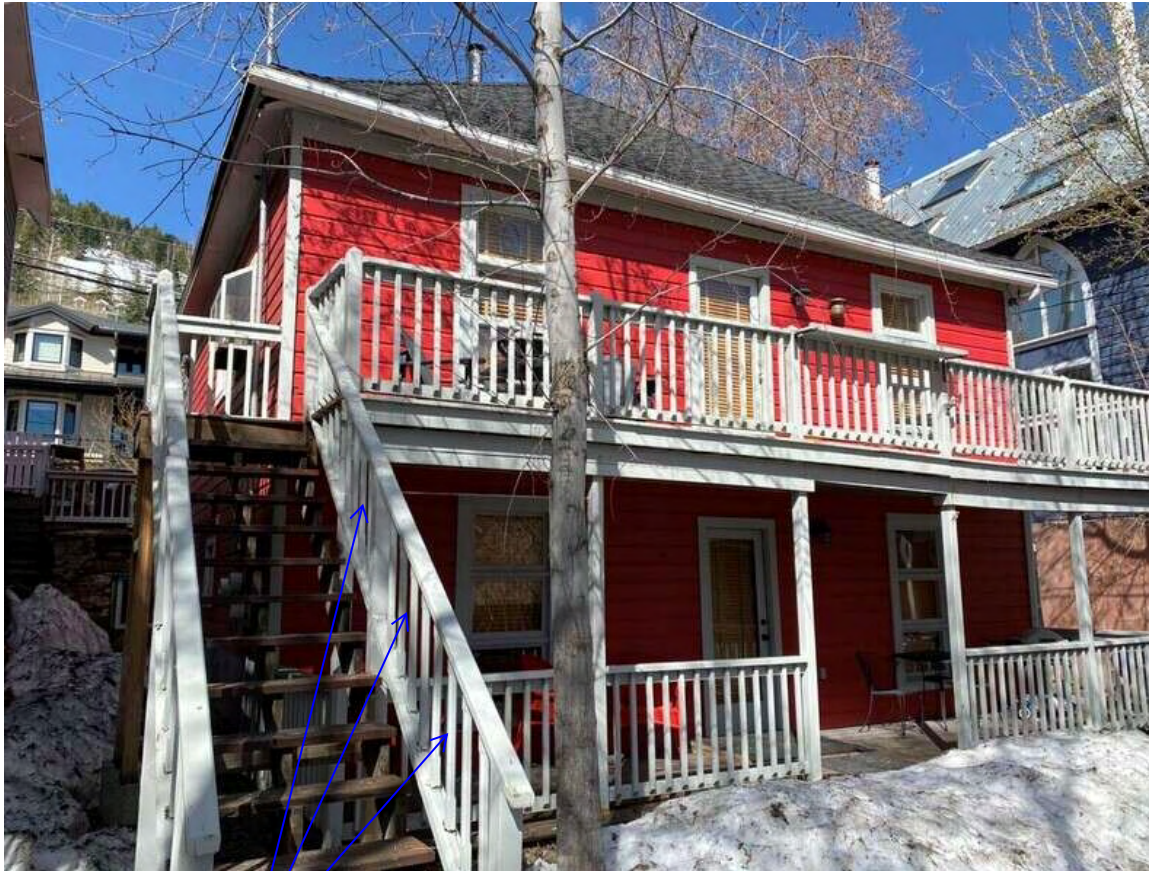
PHOTO 4: BACK ELEVATION SHOW DECK
