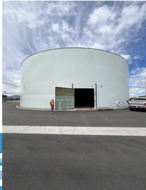
Acord Reservoir Tank
