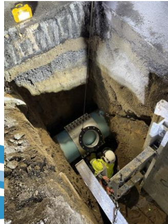
24-inch hot tap installation
