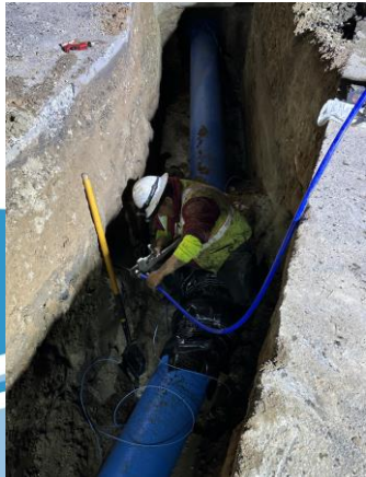
161 Service line installation
