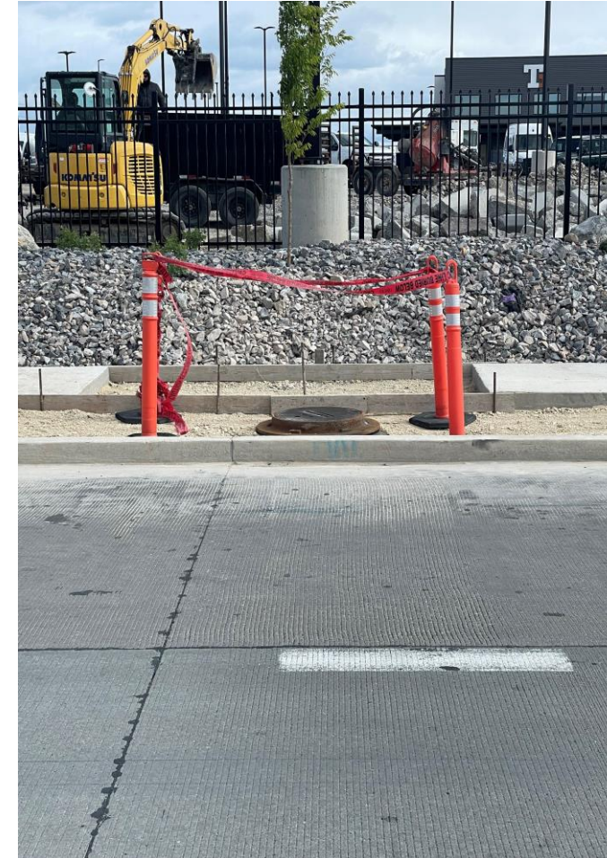
Meter relocated into park strip
