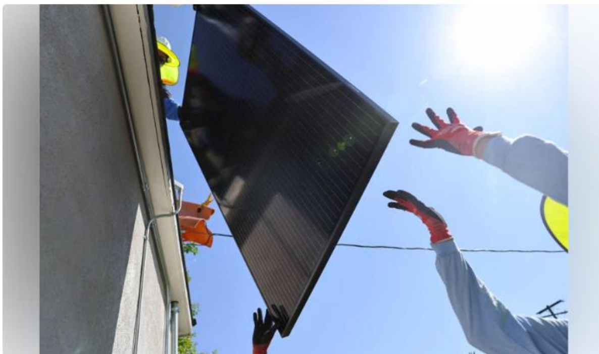
Workers hoist a solar panel on a roof in California. © Mario Tama/Getty Images
